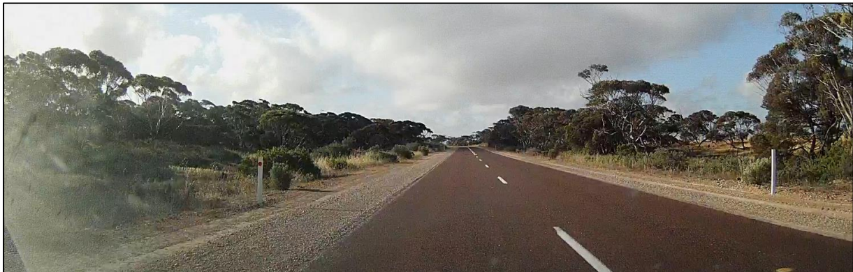
Figure 9 – Typical road environment with roadside drops, trees beyond and lack of edge lines
