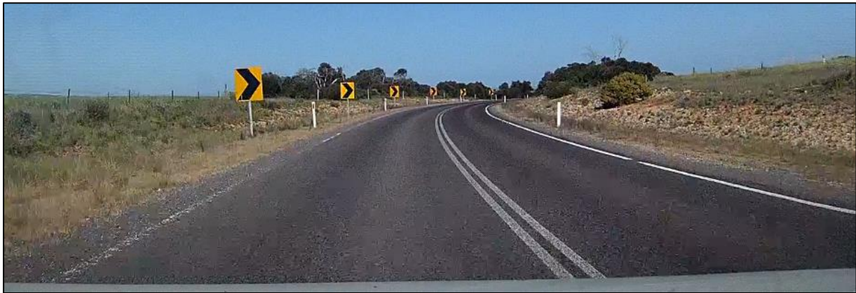
Figure 19 – Chevron Alignment Markers provide clear delineation on bends
