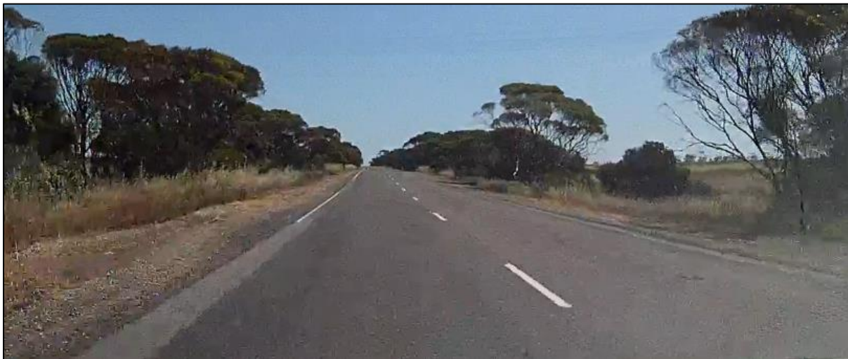
Figure 12 – Inconsistent edge line marking
