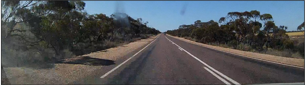
Figure 5 – Typical road environment with bitumen bleeding, roadside drops and large trees
