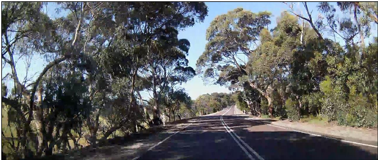
Figure 18 – Significant vegetation with large drop (left)
