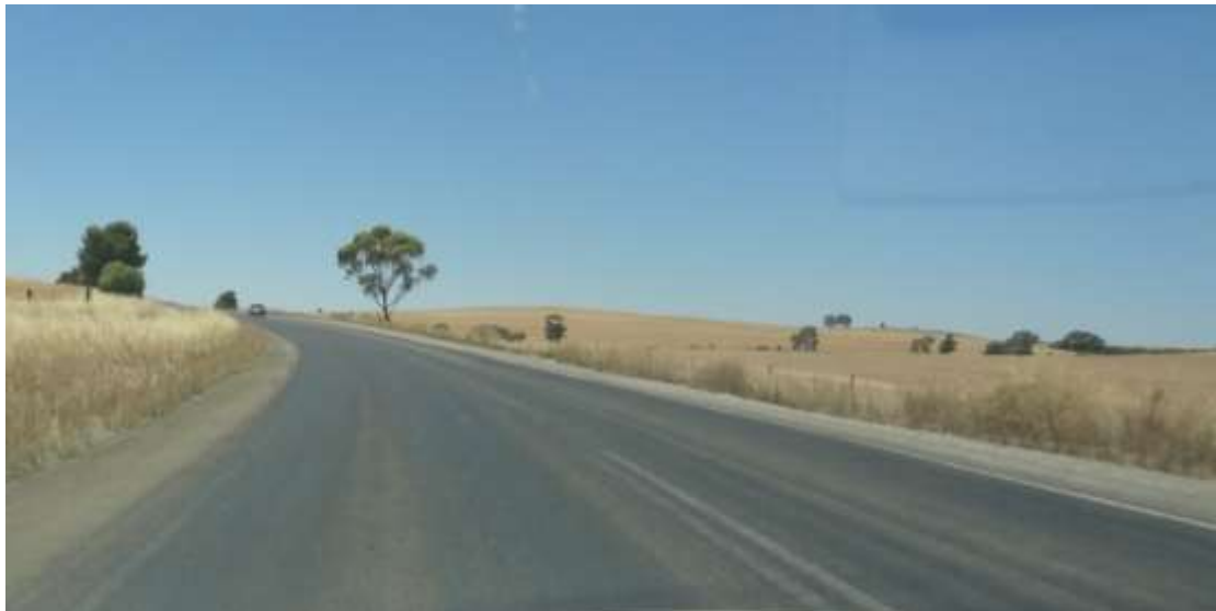
Figure 3: Aggregate loss in the road surface resulting in line markings which cannot be seen.
