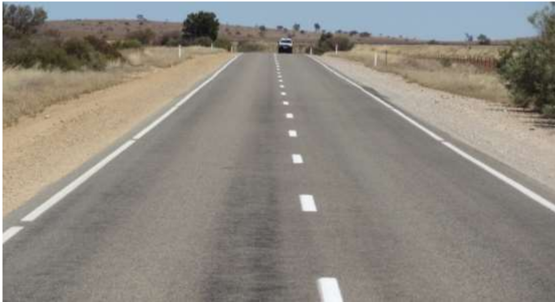
Figure 2: A section of road between the Barrier Highway and Peterborough. Surface conditions and line markings are good; however the lanes and shoulder seals are narrow.
