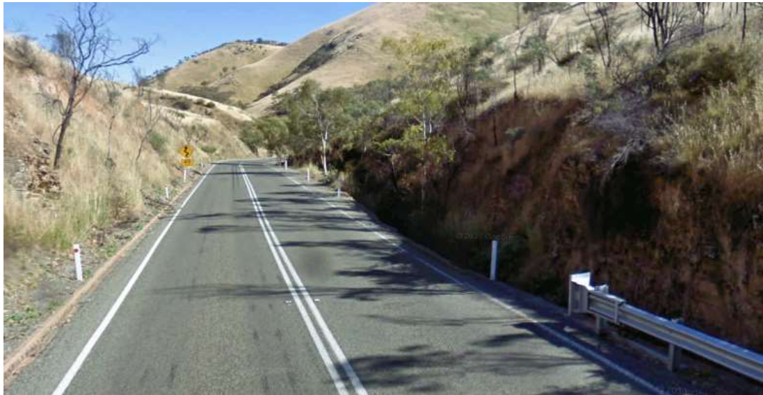
Figure 7: A section of Horrocks Pass with a large unprotected drop on the side of the road. Provided W-Beam railing does not fully protect this hazard. Suggested speed sign reads 45km/h (Google Street view 2009).
