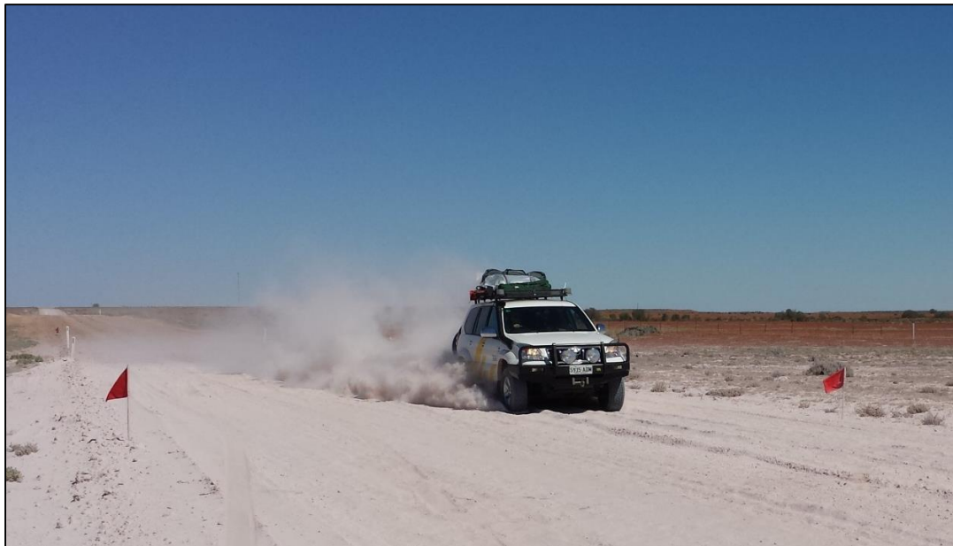
Figure 10 – Bull dust holes have been marked with red flags. They create a rollover risk and severely restrict sight distance for any vehicles following or passing the vehicle travelling through them.
