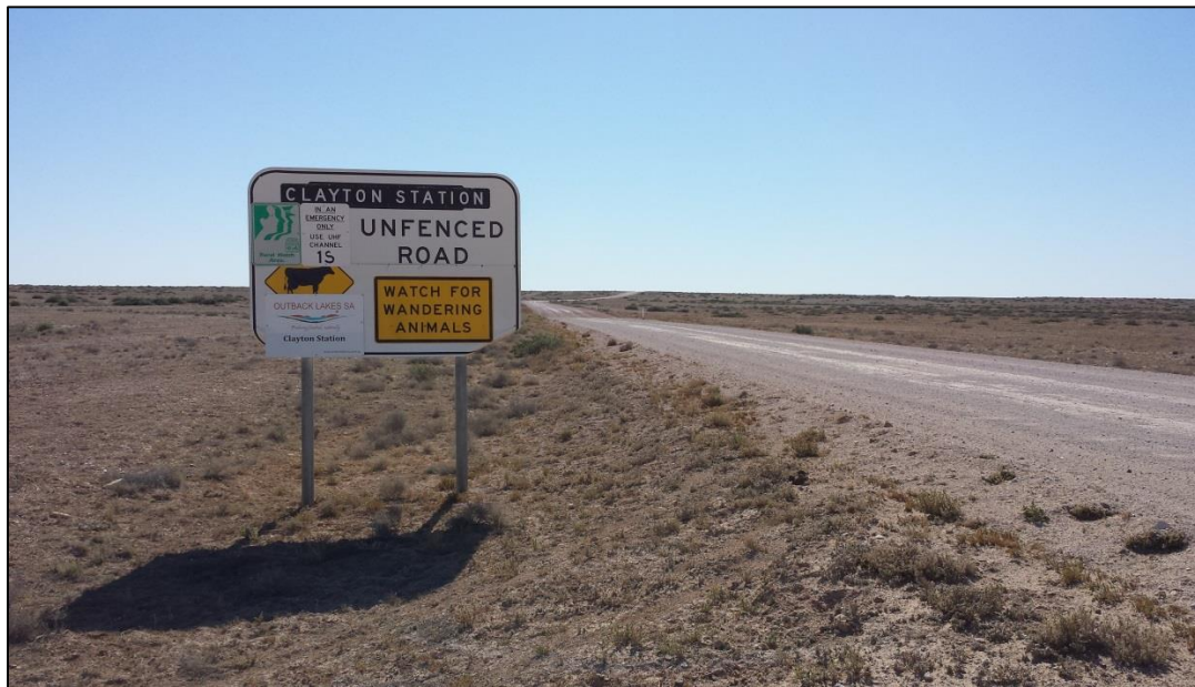
Figure 8 – Additional unauthorised signs have made this warning sign cluttered and difficult for the motorist to read.
