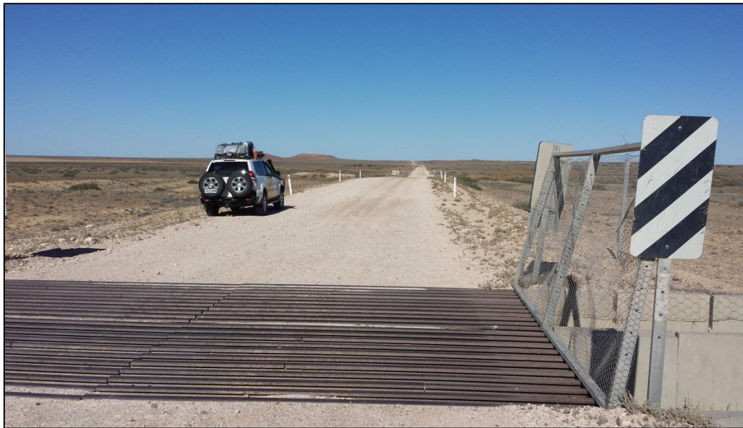
Figure 9 – Hazard boards have been provided at grids where the road narrows but little protection is offered from the drops on either side.
