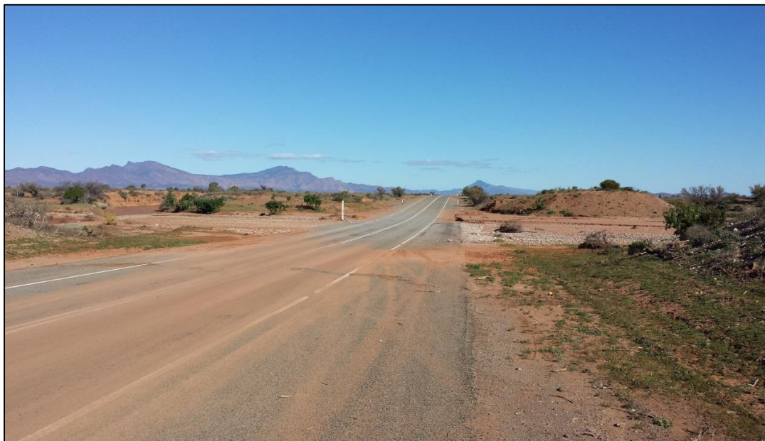
Figure 4 – Sediment has washed across the road and could create a skid hazard under wet conditions.
