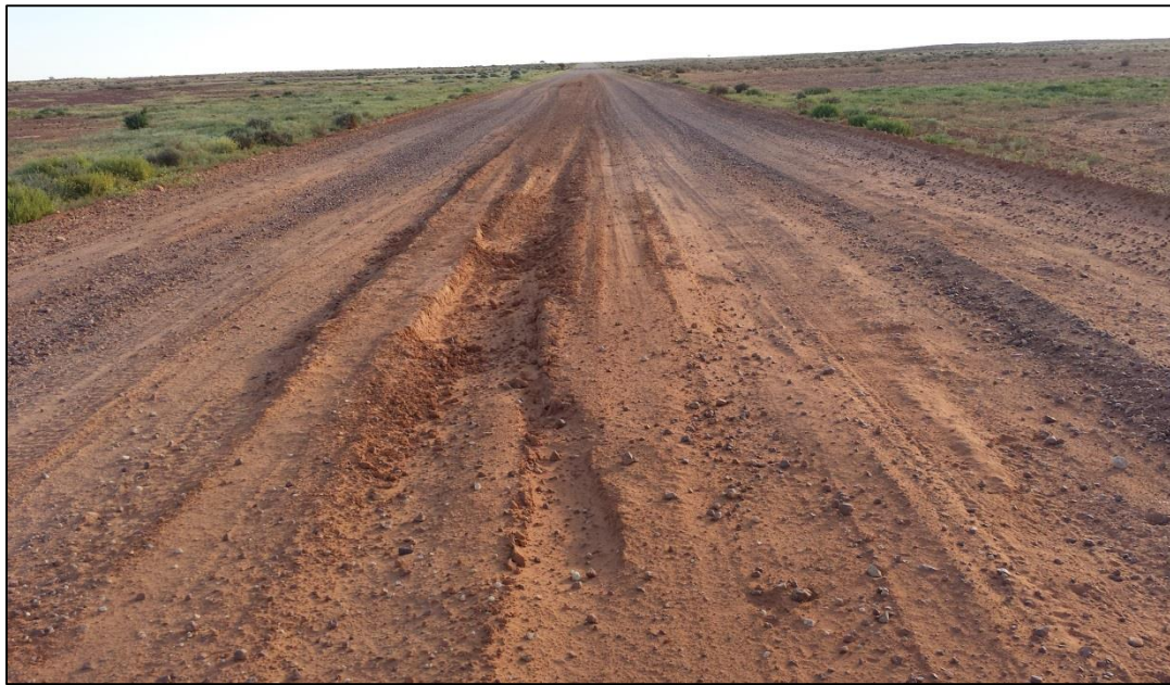
Figure 16 – Bad rutting recorded along the track.
