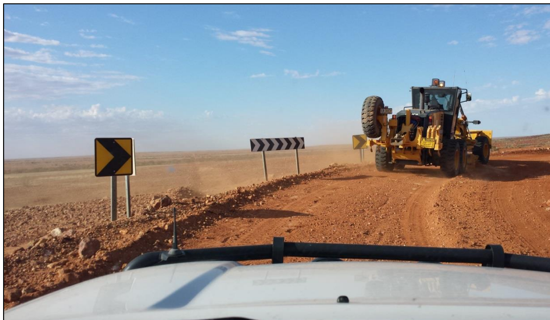
Figure 15 – The survey team encountered graders undertaking maintenance along the track at a number of locations.
