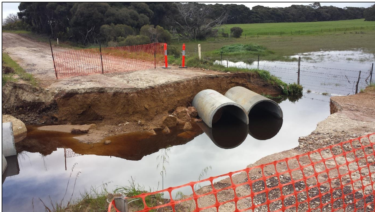
Figure 3 – Flood water completely washed away a section of Old South Coast Road, including the large concrete storm pipes.
