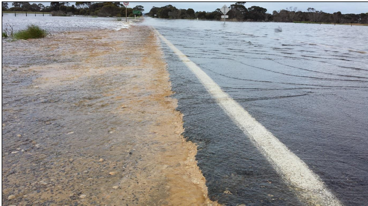
Figure 2 – Water eroding the pavement and shoulder on Hog Bay Road near the intersection with Playford Highway.
