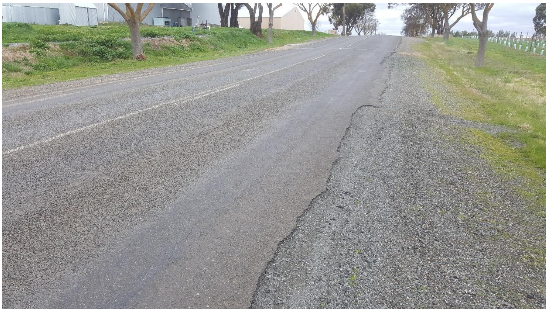
Figure 52: Crumbling edges are a significant issue in some sections of Seppeltsfield Road
