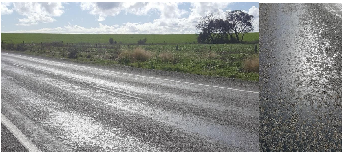
Figure 32: Example of the polished surface and bleeding along the majority of Horrocks Highway.
