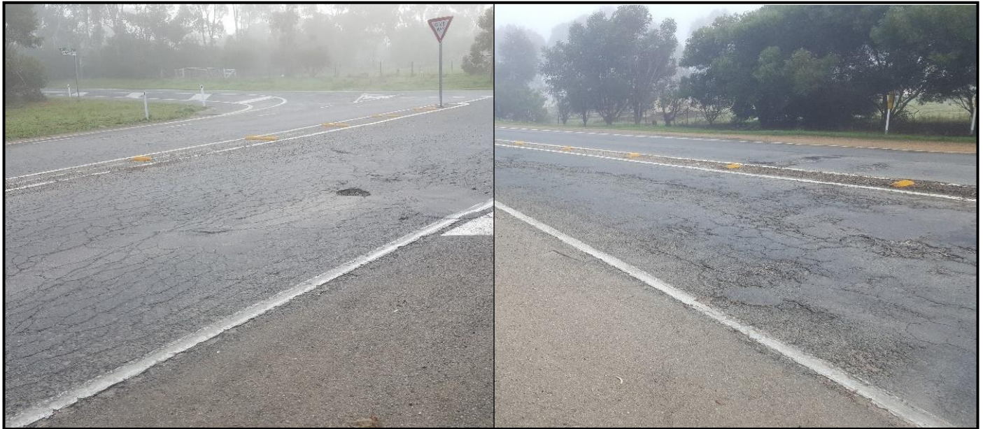
Figure 57 Cracking and Potholes on Kentish Road
