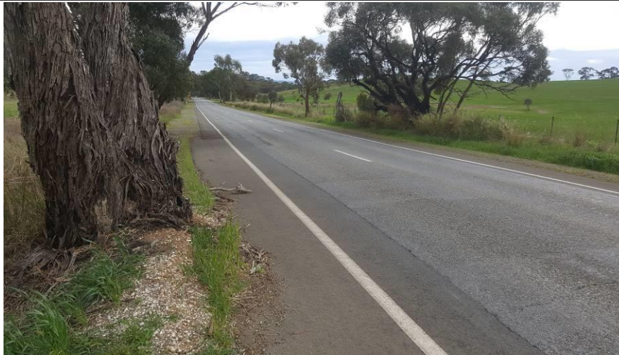
Figure 49: Significant gum tree located very close to Greenock Road posing a significant hazard
