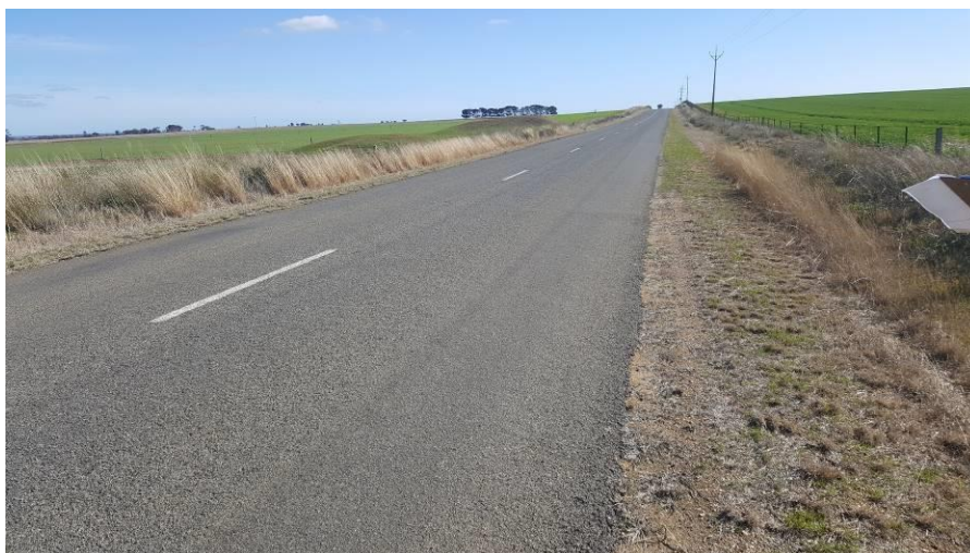
Figure 47: Templers Road (Wasleys-Templers) lacks edge lines and sealed shoulders
