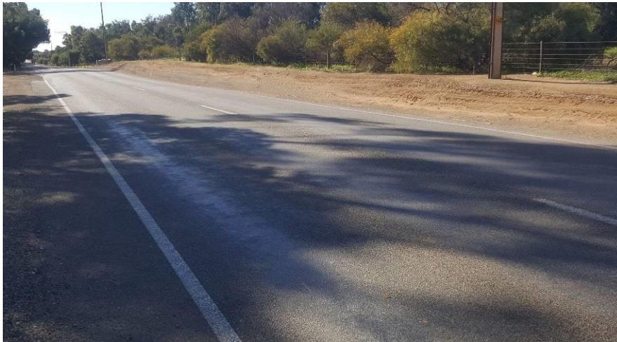
Figure 58: Undulations and surface polishing on Mudla Wirra Road south of Roseworthy Campus
