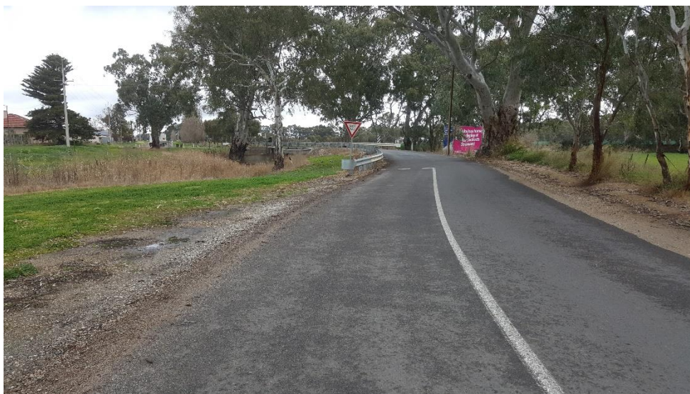
Figure 63: Visibility is very poor for southbound vehicles crossing the bridge.
