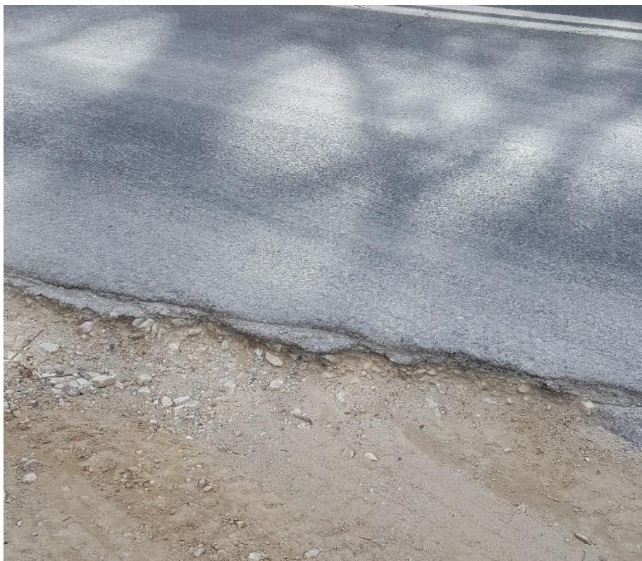
Figure 50: 100mm drop off at the intersection of Parbs Road and Sir Condor Laucke Way
