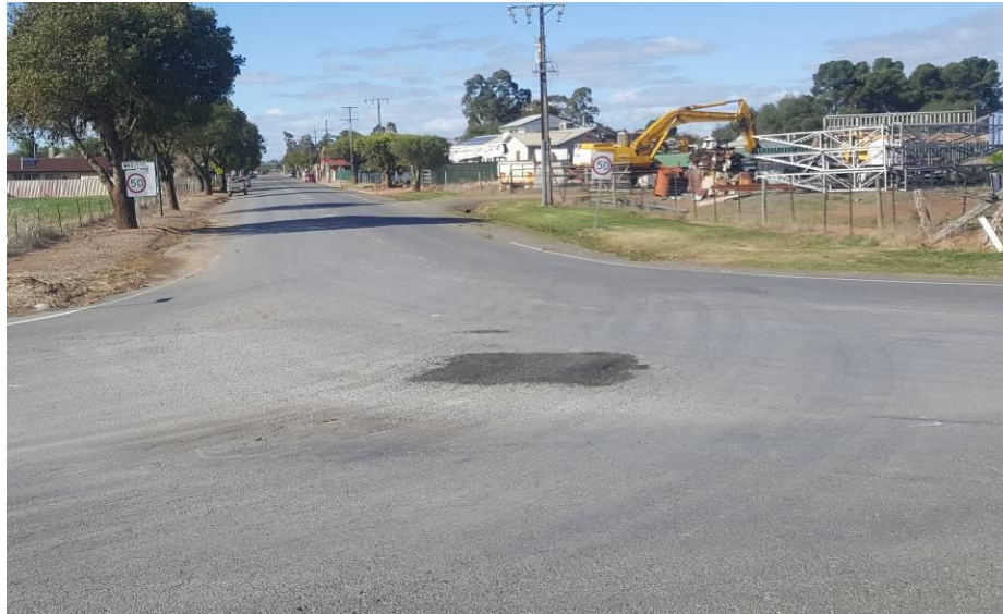
Figure 59: Line marking is barely visible at the intersection with Annie Terrace
