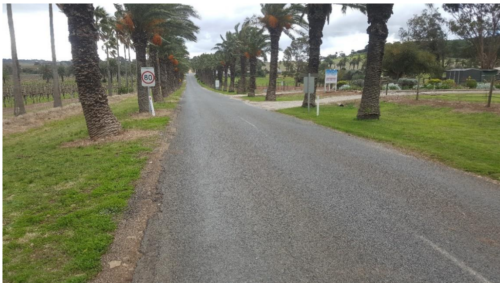
Figure 53: The 80km/h speed limit increases the risk of serious crashes involving the palm trees on Seppeltsfield Road
