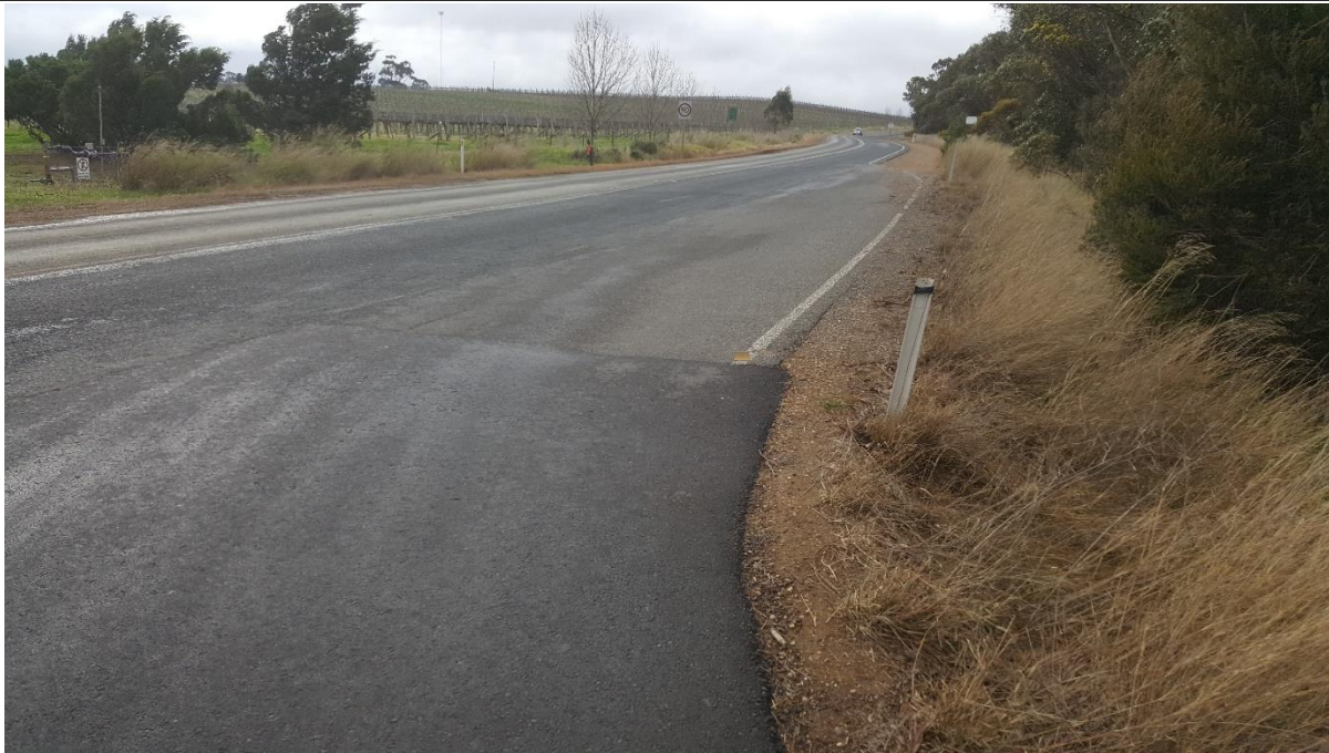
Figure 39: missing and faded line marking at the intersection of Rosedale Road
