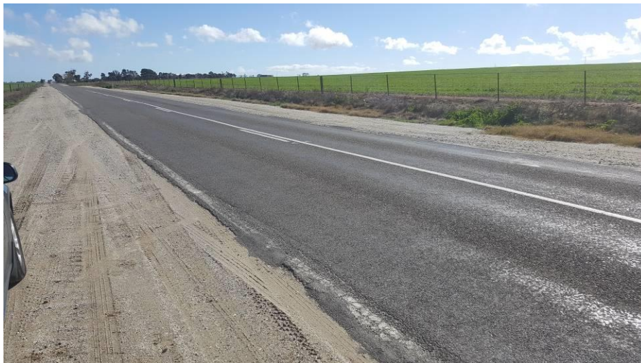
Figure 46: Poor edges and a lack of unsealed shoulders were some of the primary concerns on Owen Road
