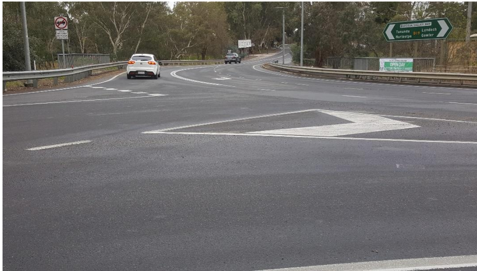
Figure 43: The left turn slip lane onto Gomersal Road (foreground) causes some confusion with priorities
