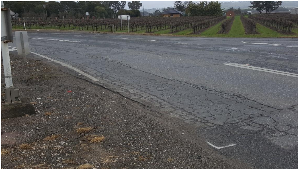
Figure 45: The surface at this intersection is in very poor condition
