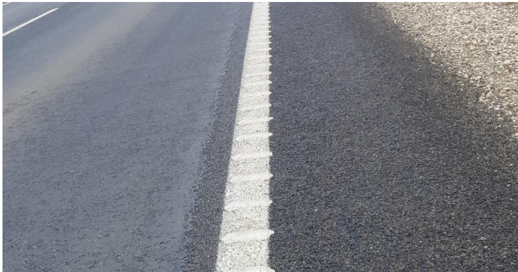
Figure 37: A highly polished carriageway next to recent installation of ATLM and shoulder widening
