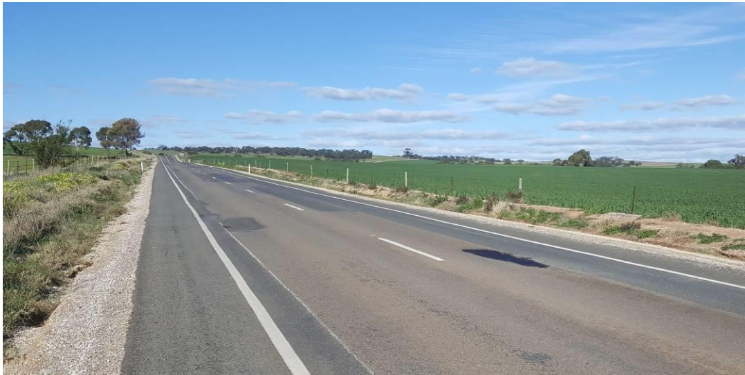
Figure 48: Uneven and patched surface at the eastern end of Daveyston Road.
