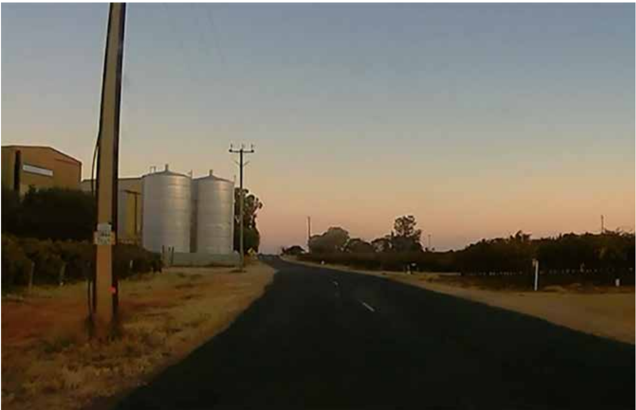
Stobie poles were located very close to the road and poorly delineated
