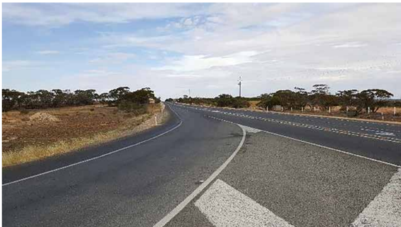
The acceleration lane at the Stanitzki Road/Bookpurnong Road intersection is too short for slower vehicles to safely merge
