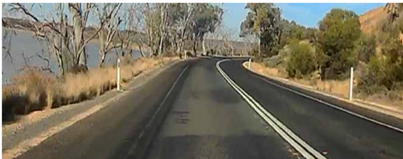
Faded edge lines around curves were common, as were steep drop offs and fixed objects in the clear zone as pictured
