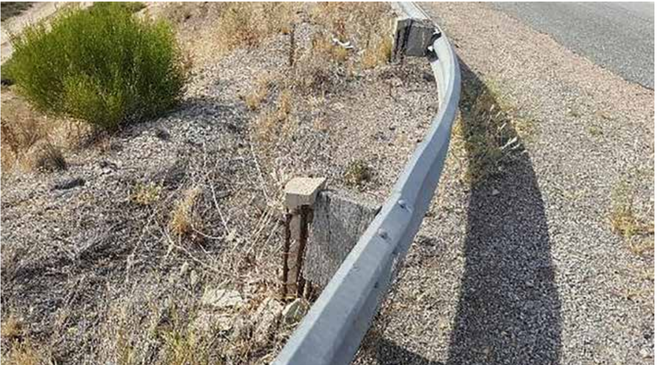
W-beam barrier supports at this intersection are in poor condition
