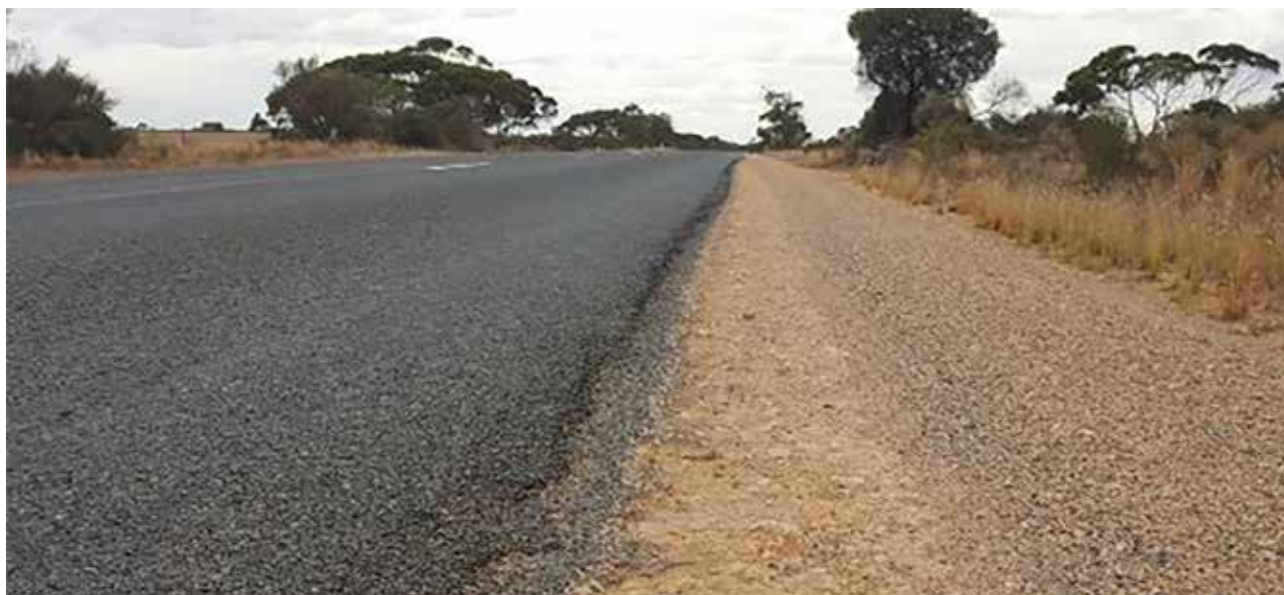
Edge drop off was prevalent in a number of locations
