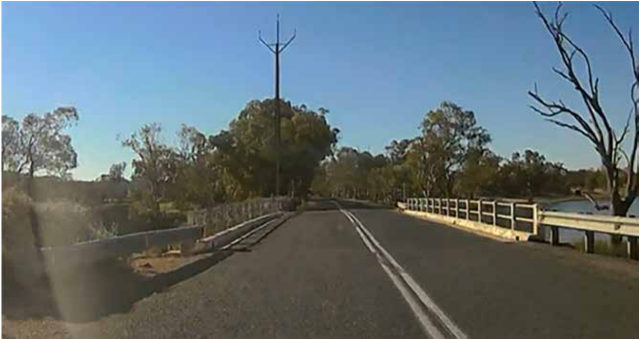
Width markers are not installed to delineate the width of Nappers Bridge
