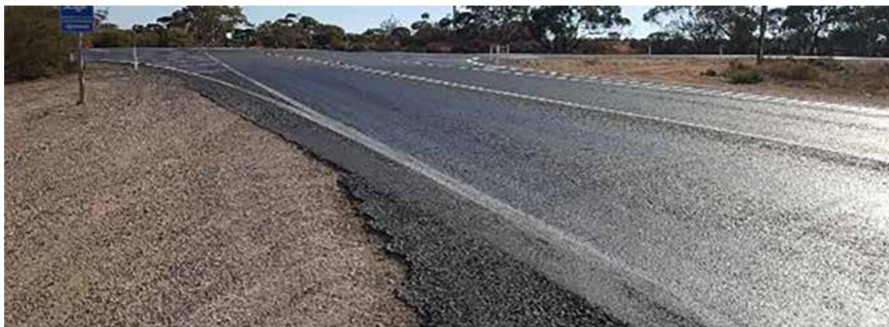
The highly polished surface on Kingston Road on approach to Sturt Highway is likely to perform poorly in wet weather
