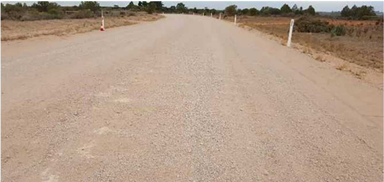
Corrugations on sections of the road, with the protruding rock bed a potential cause of tyre blowouts
