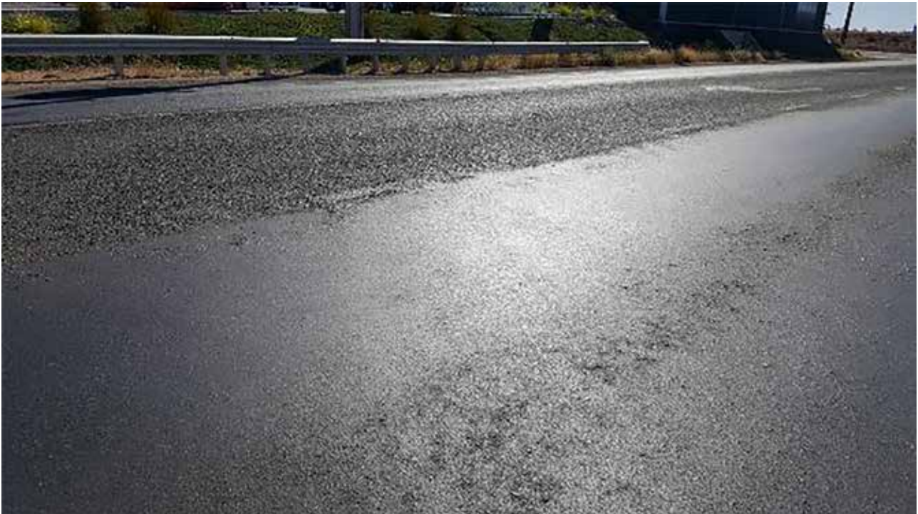
Slippery pavement and very faded line marking is a major safety concern near Bunnings in Berri
