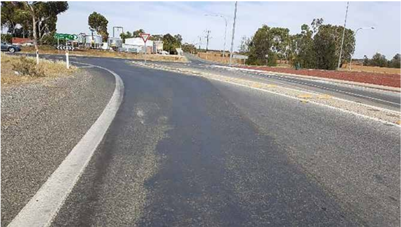
A highly polished surface and faded line marking increase the risk at this intersection
