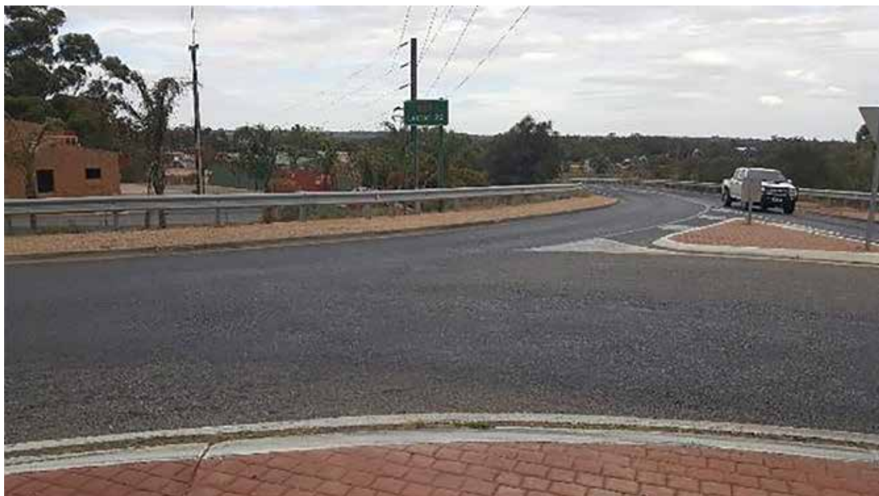
The exit curve of the roundabout in Berri is challenging for heavy vehicles to negotiate.
