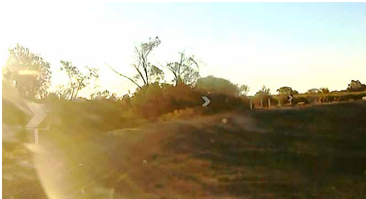
Unidirectional hazards markers were incorrectly used around a number of curves
