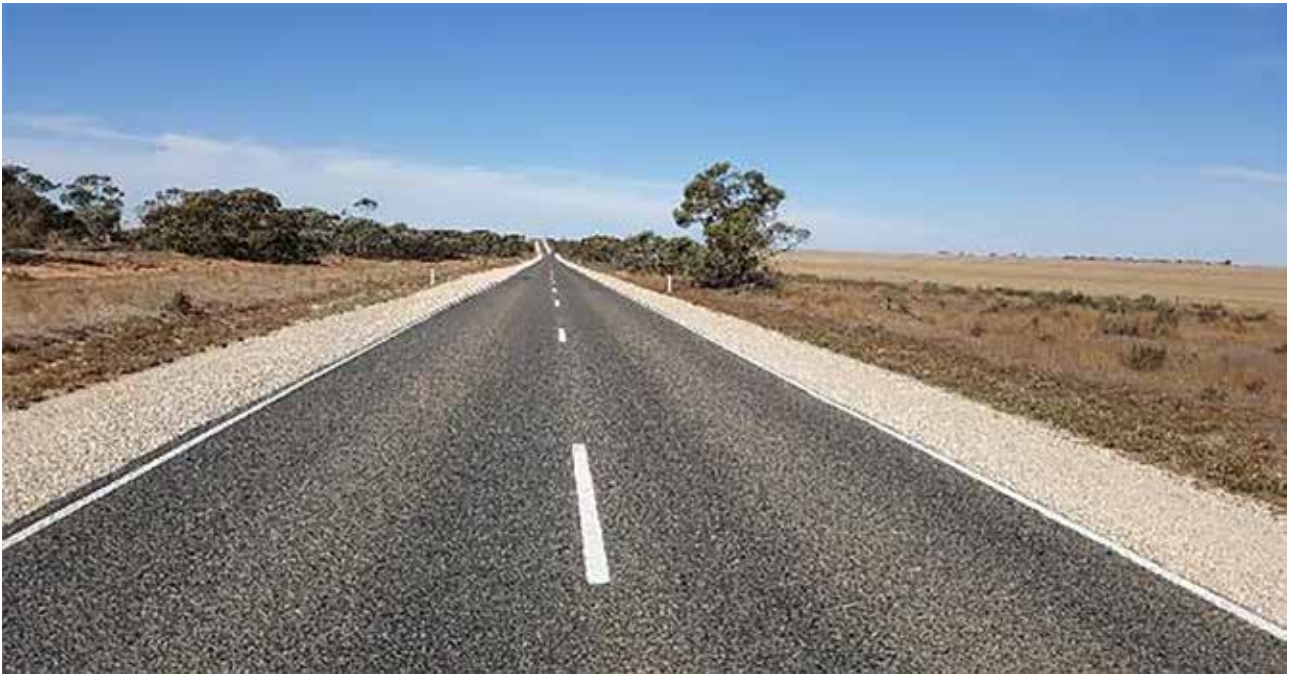
Ten kilometres of edge lines narrowed the lanes however delineated the road edges
