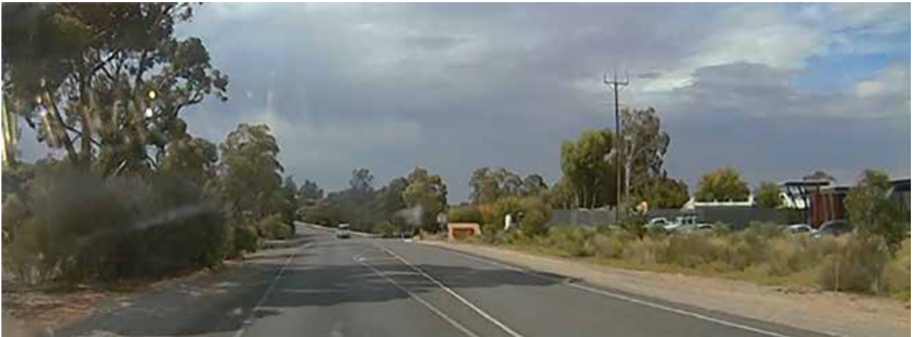
Faded line marking in the vicinity of Edmondson Road
