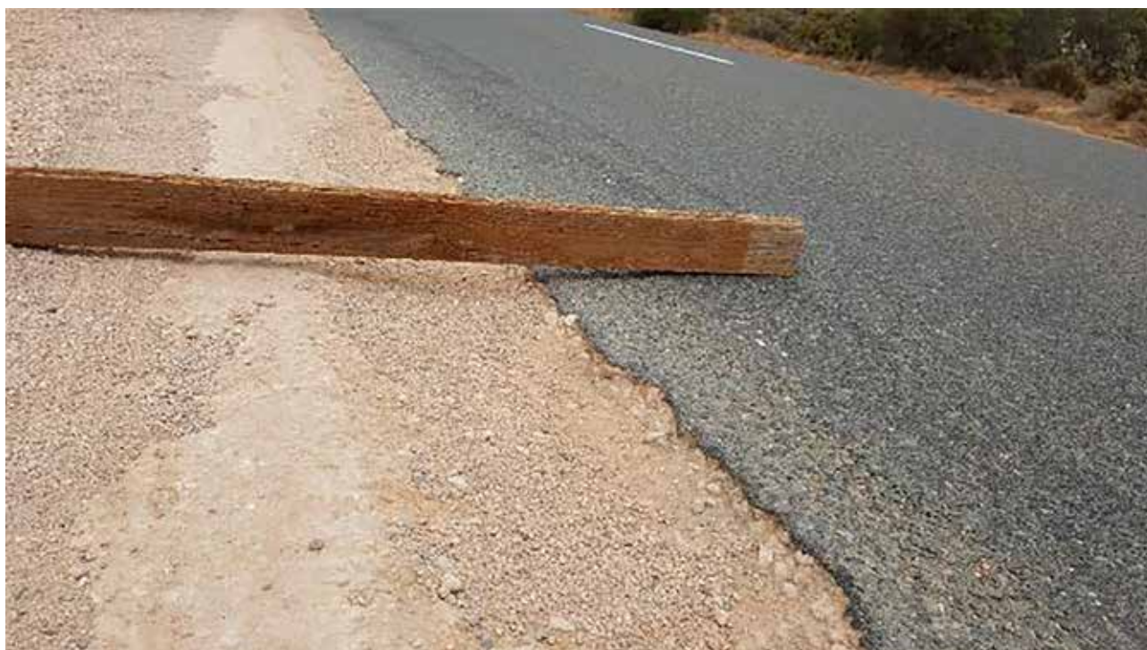
Drop-offs were measured between 50-100mm along most of Stanitzki Road
