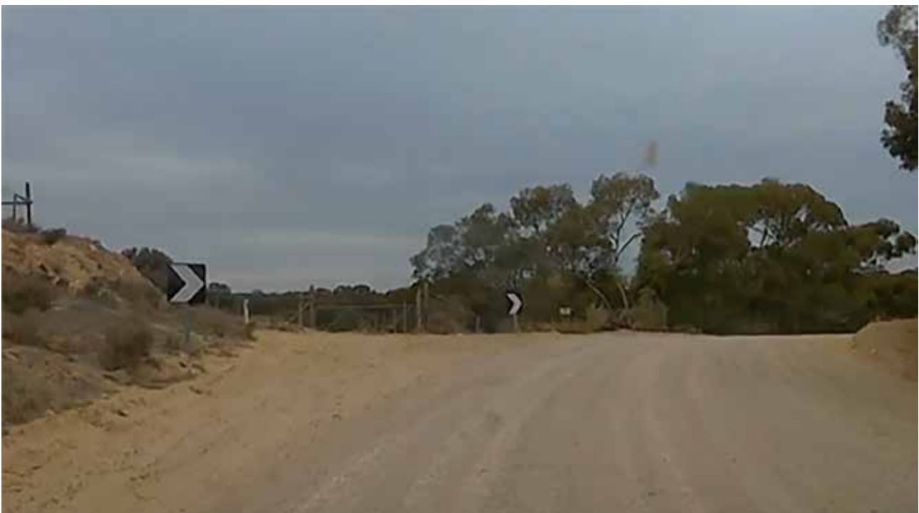
Unidirectional hazard marker boards were incorrectly installed to delineate substandard curves.
