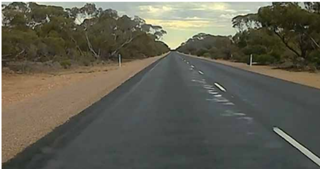
Water ponding on the surface after light rainfall
