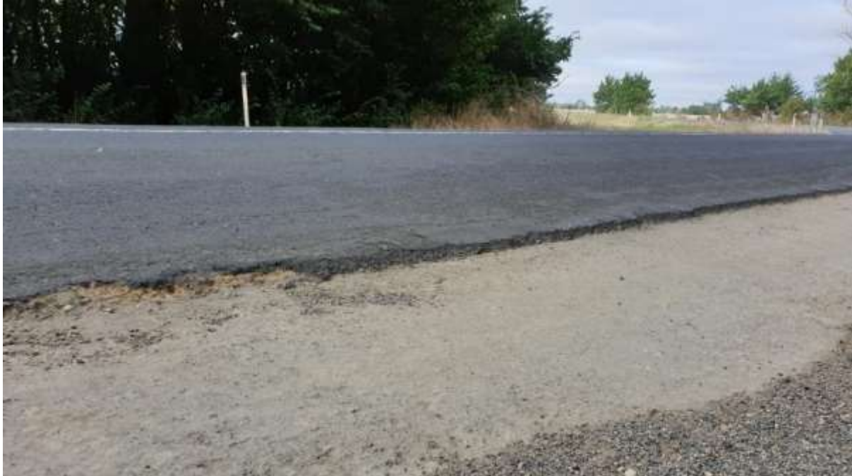
Broken edges and drop-offs on the narrow section between Penola and Wattle Range
