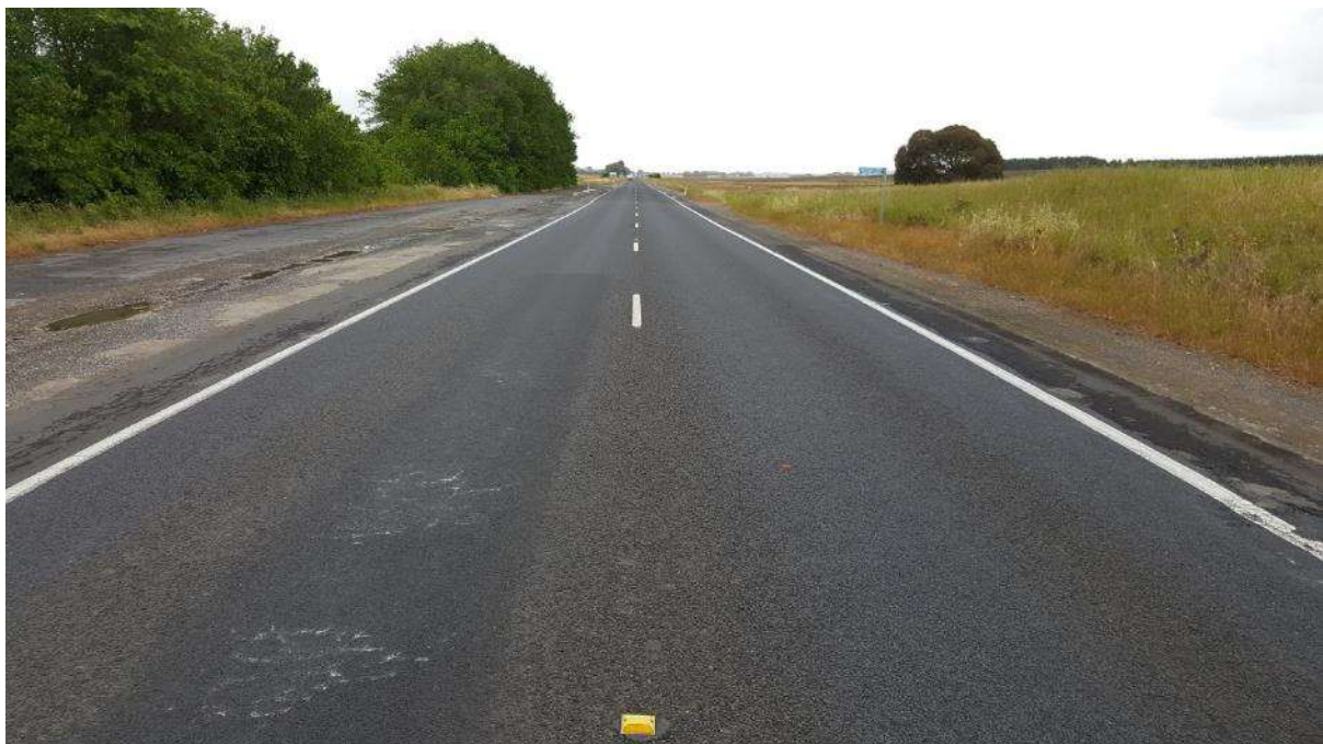
Rutting and cracking in the wheel paths in Mingbool
