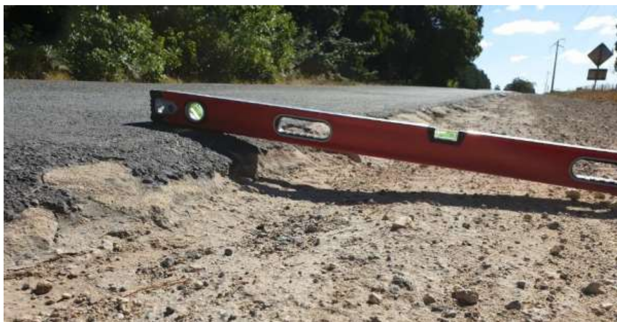
Edge break up and drop off on the southern end of Kangaroo Flat Road
