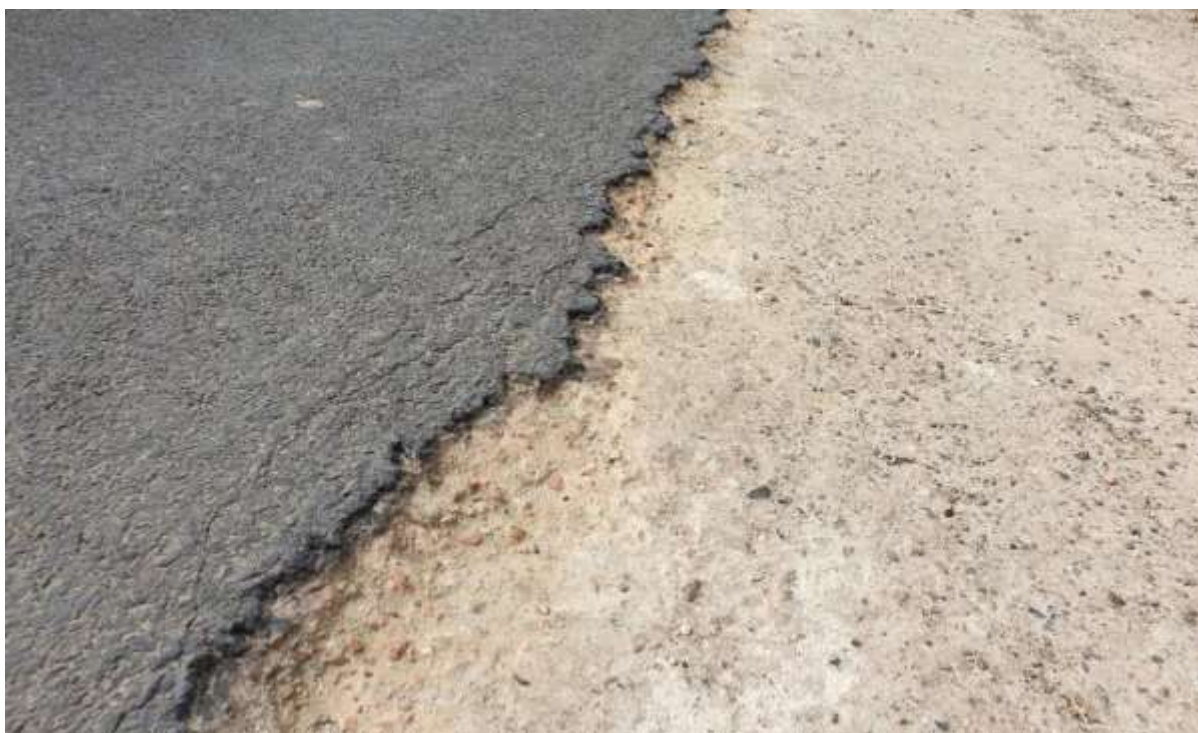
Broken edges and drop off on Tillers Road
