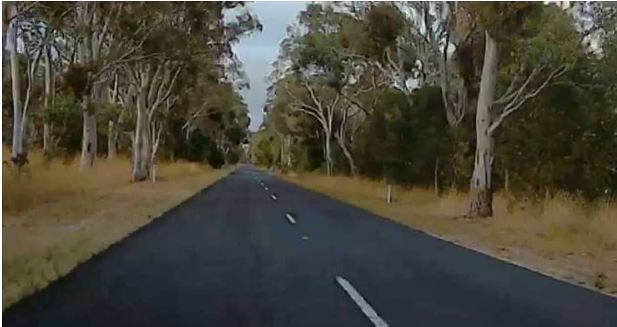
Trees growing in close proximity to the road edges pose a substantial risk in run off road crashes.
