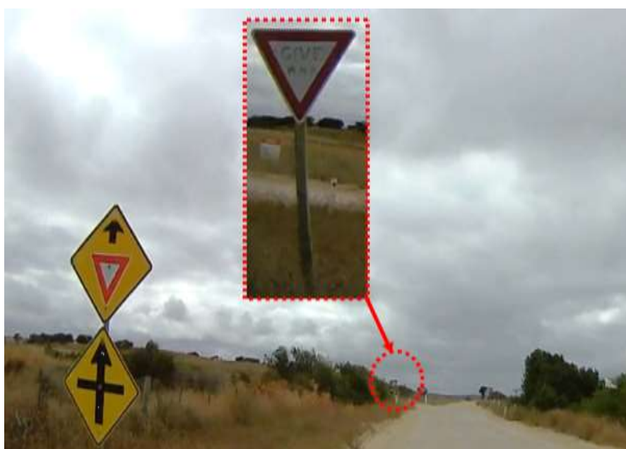
Conflicting 'give way ahead' and intersection warning signs on Nora Creina Road, and faded give way sign (inset)
