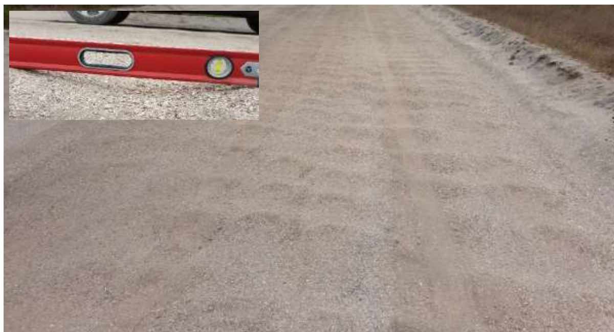
Corrugations and a slippery surface are the primary issues noted on Bog Lane
