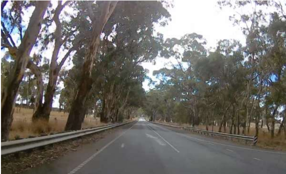
Barrier protection to combat crashes into trees along Wimmera Highway
