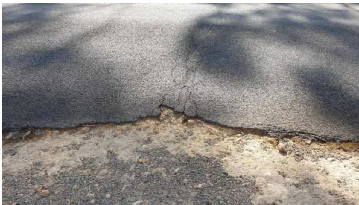
Poor condition of road edges and unsealed shoulders on Casterton Road
