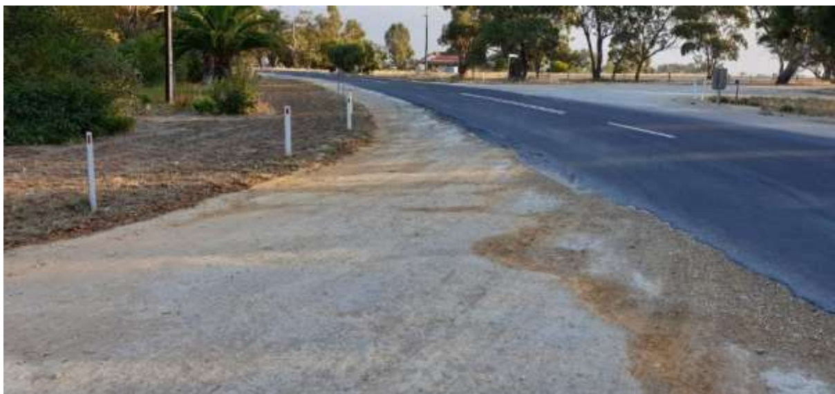
Sight distance to the north from Stott Road is poor
