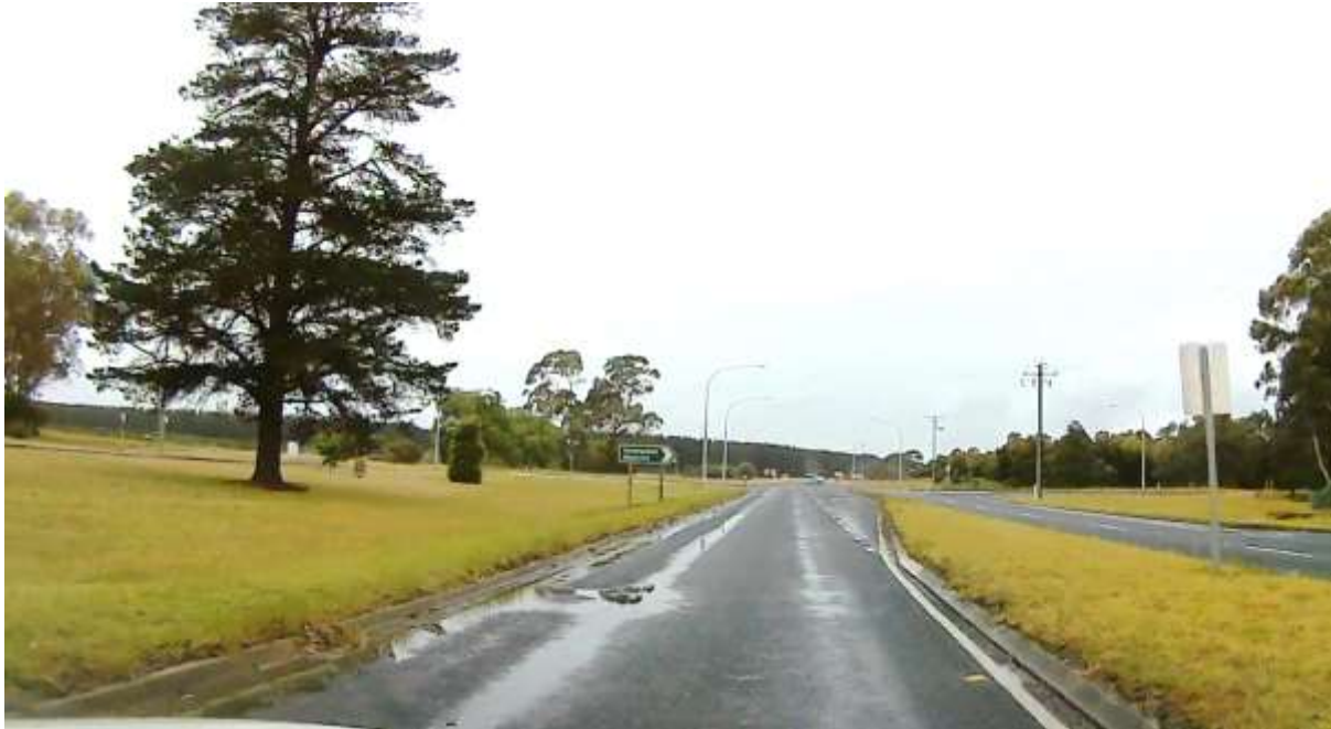
Ruts causing ponding in Nangwarry
