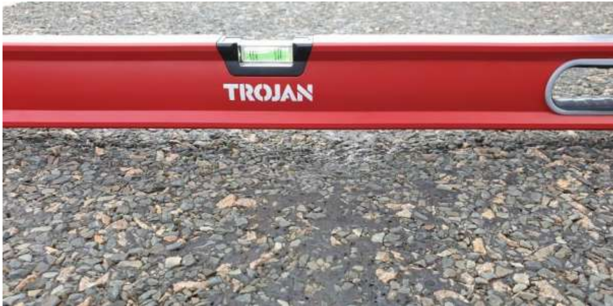
Rutting is prevalent on Ngarkat Highway
