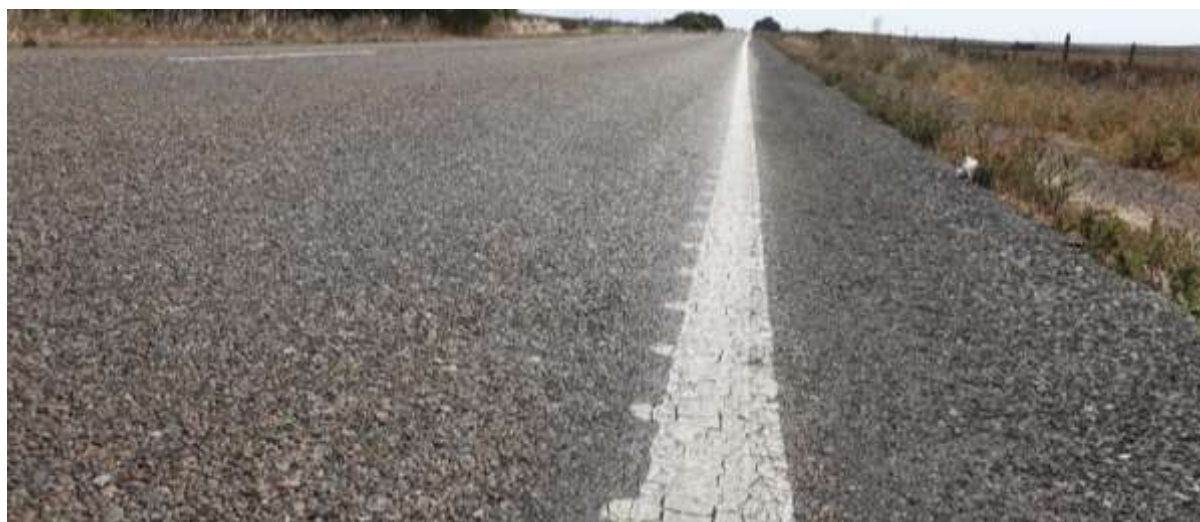
ATLM edge lines have completely worn away for most of Princes Highway between Tailem Bend and Meningie
