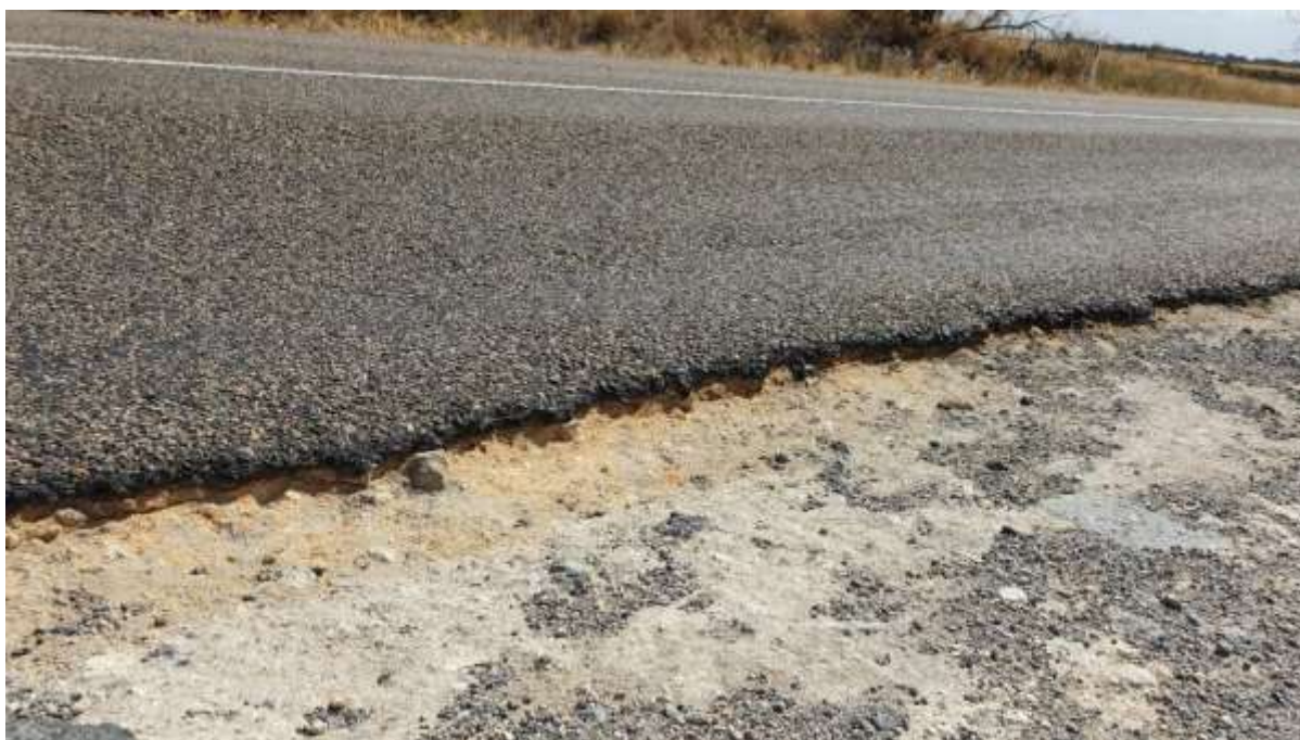
Breaking edges and associated edge drop-off persistent along Ngarkat Highway
