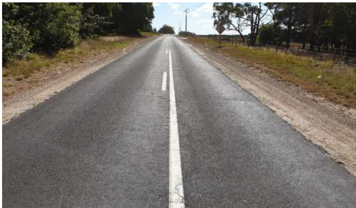
Kangaroo Flat Road is very narrow with a seal width of 5.0m measured
