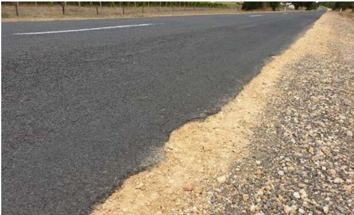
Edge drop off and breakup between the Southern Ports and Princes Highways.
