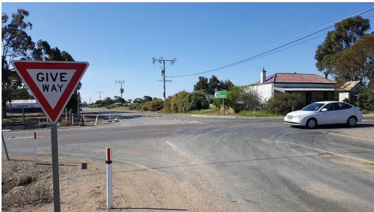
Line marking at the intersection with Copper Coast Highway and Upper Yorke Road is deteriorated
