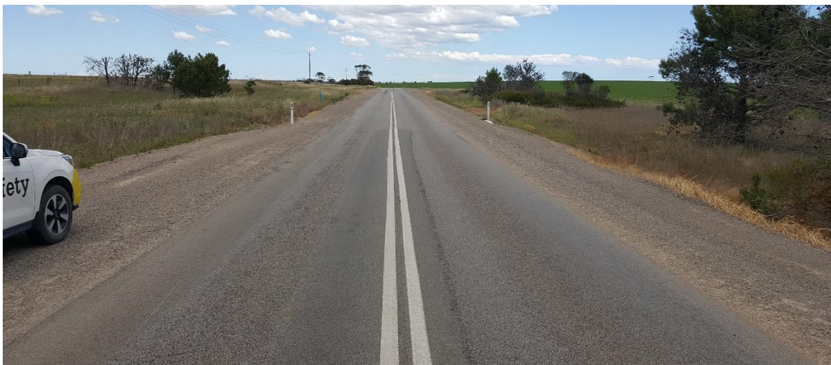
A very narrow carriageway and deteriorating surface are the primary issues between Maitland and Minlaton
