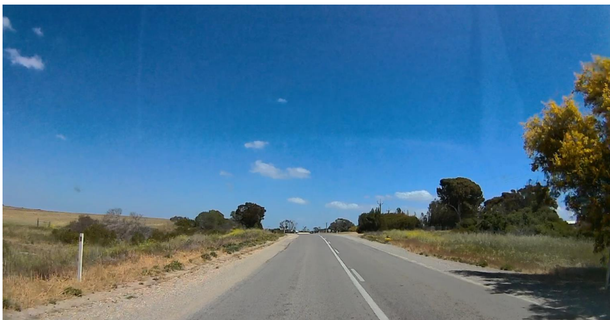
Vehicles stopped on the road turning right may be concealed by the of crest and left hand curve combination (150m north of the intersection, looking south)
