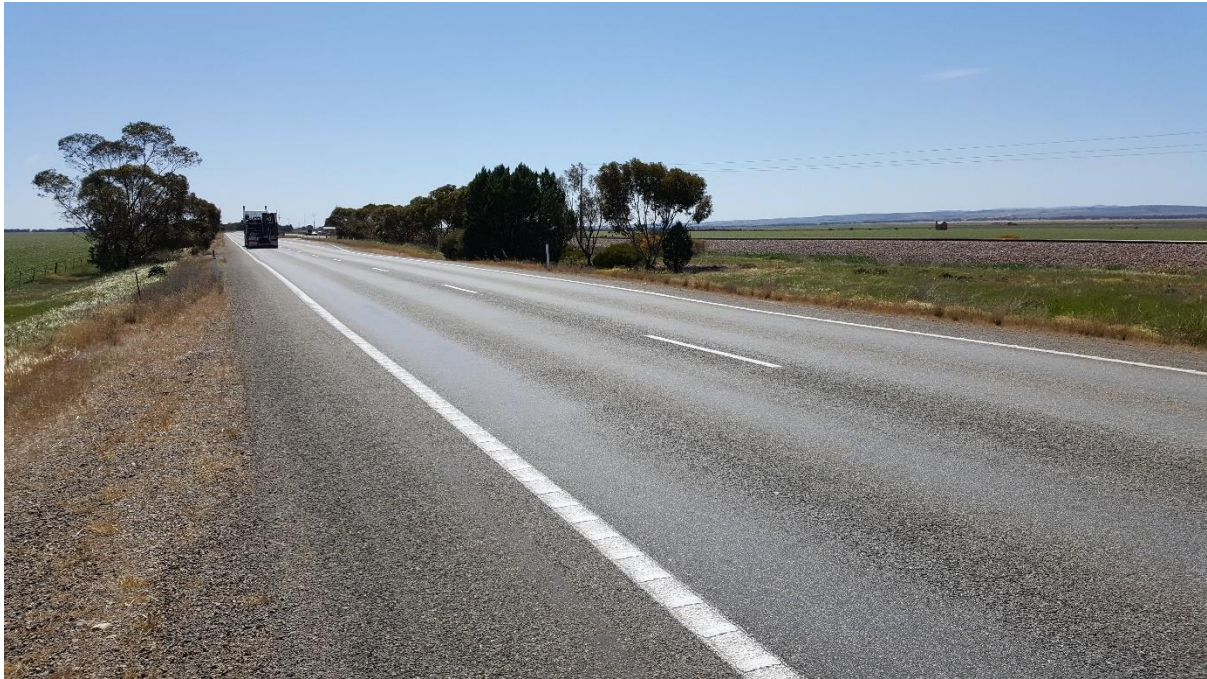
Road geometry on Augusta highway is good for a two-lane two-way road (polishing in the wheel paths is evident)
