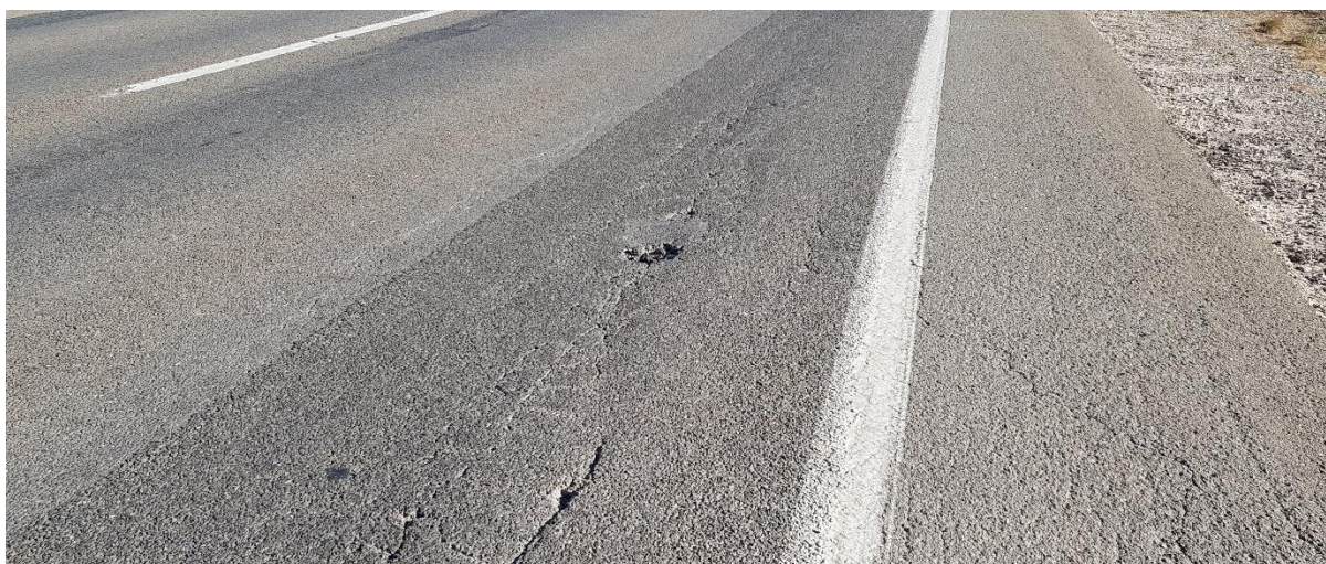
Cracking in the ruts is leading to the formation of potholes when water builds up
