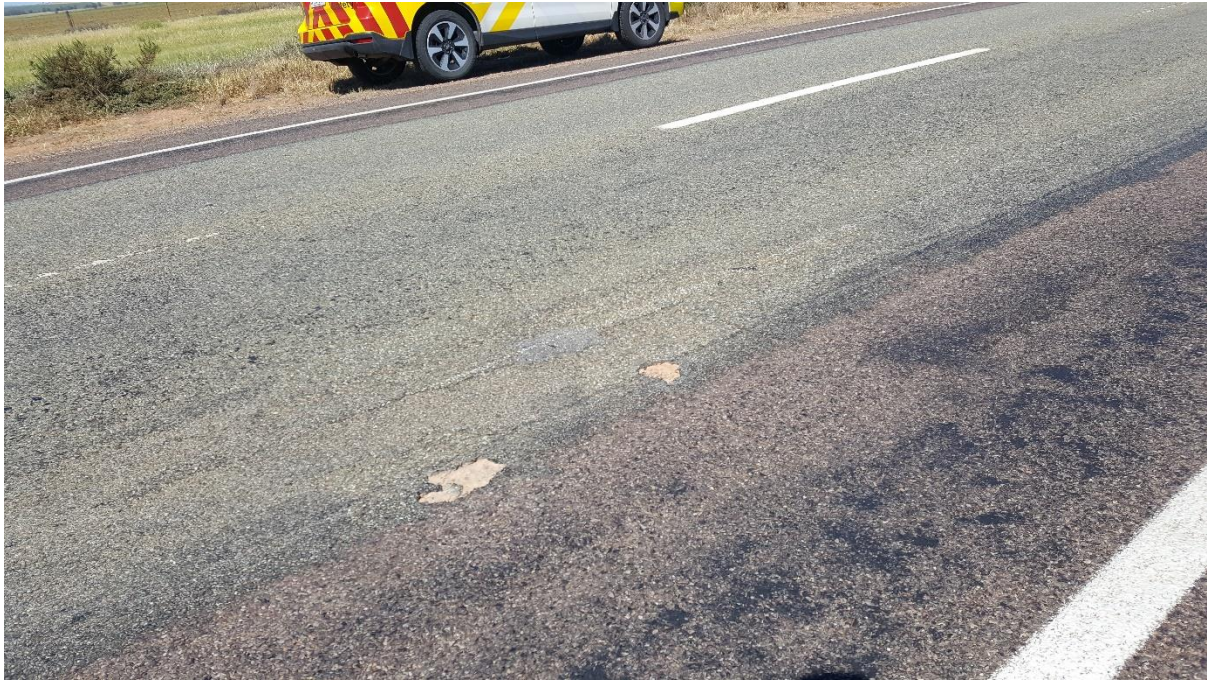
Potholes forming on the join between the shoulder seal and previous seal
