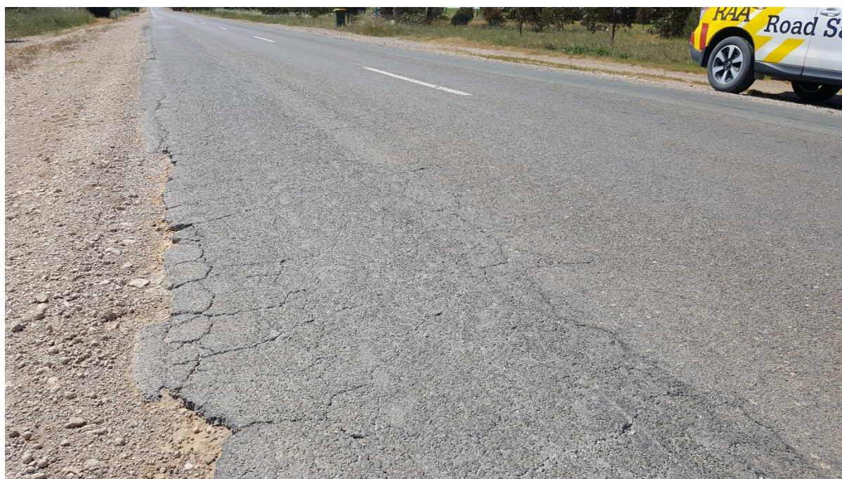
Failing section of Harry Butler Road (northbound lane)
