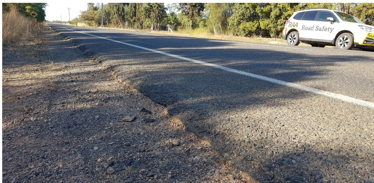
Substantial edge drop-offs were prevalent south of the Korunye rail crossing.
