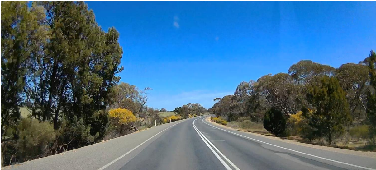
Unprotected drop-off and dense roadside vegetation east of Balaklava
