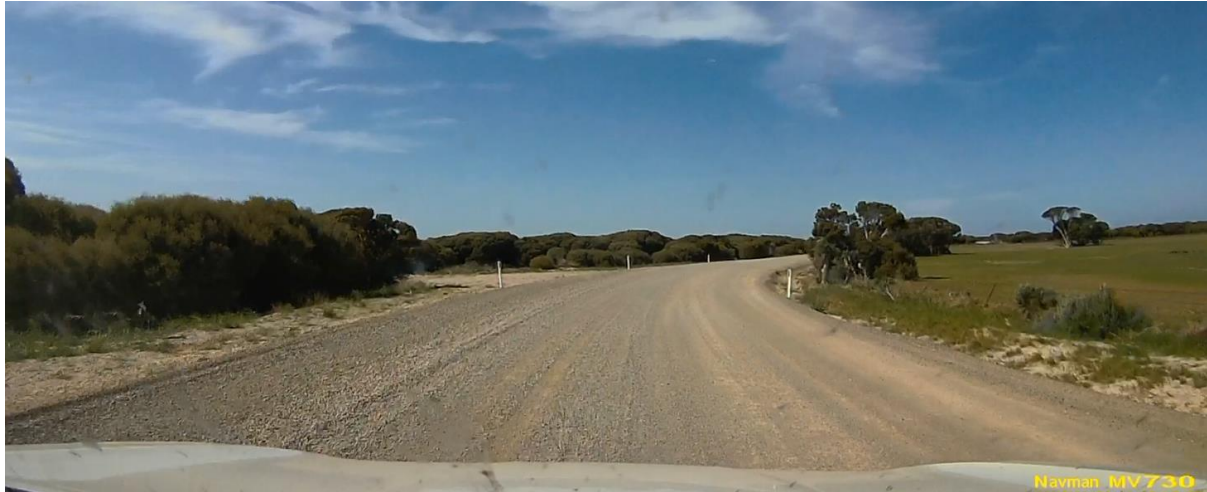
Ridges of loose material are prevalent on some sections of South Coast Road
