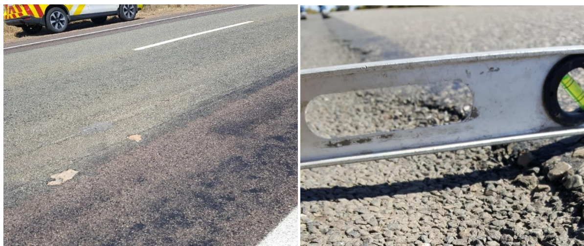
Examples of poor joins between shoulder seal and existing pavement
