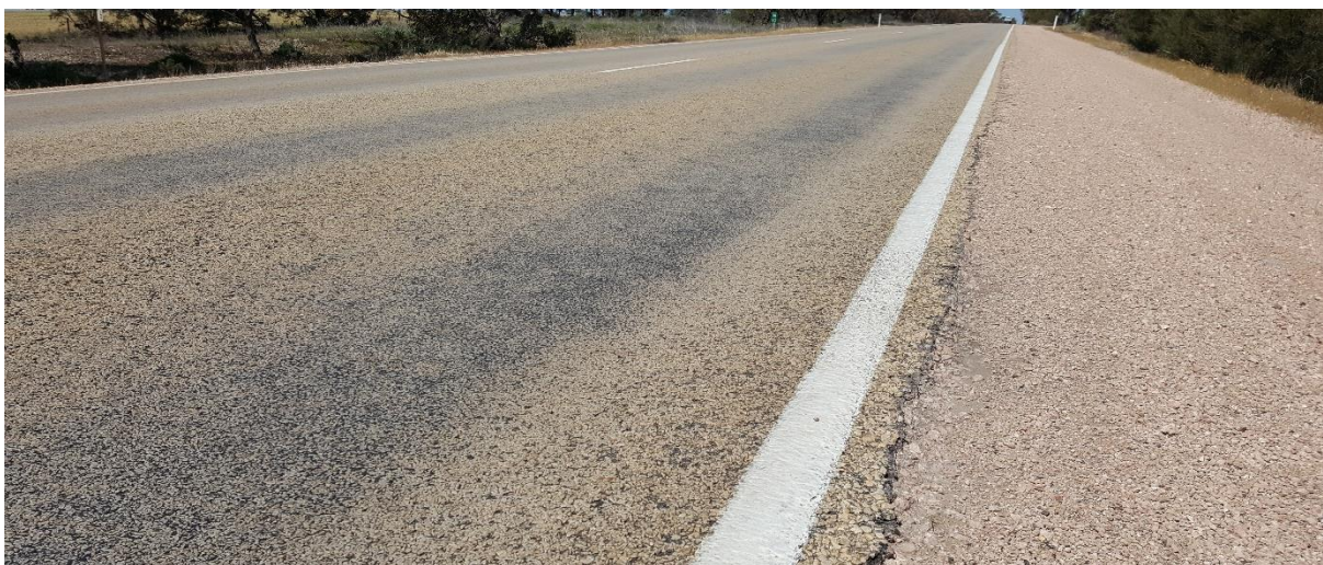
A typical section of Spencer Highway (Wallaroo – Moonta) with wide lanes, narrow shoulder seal and ruts
