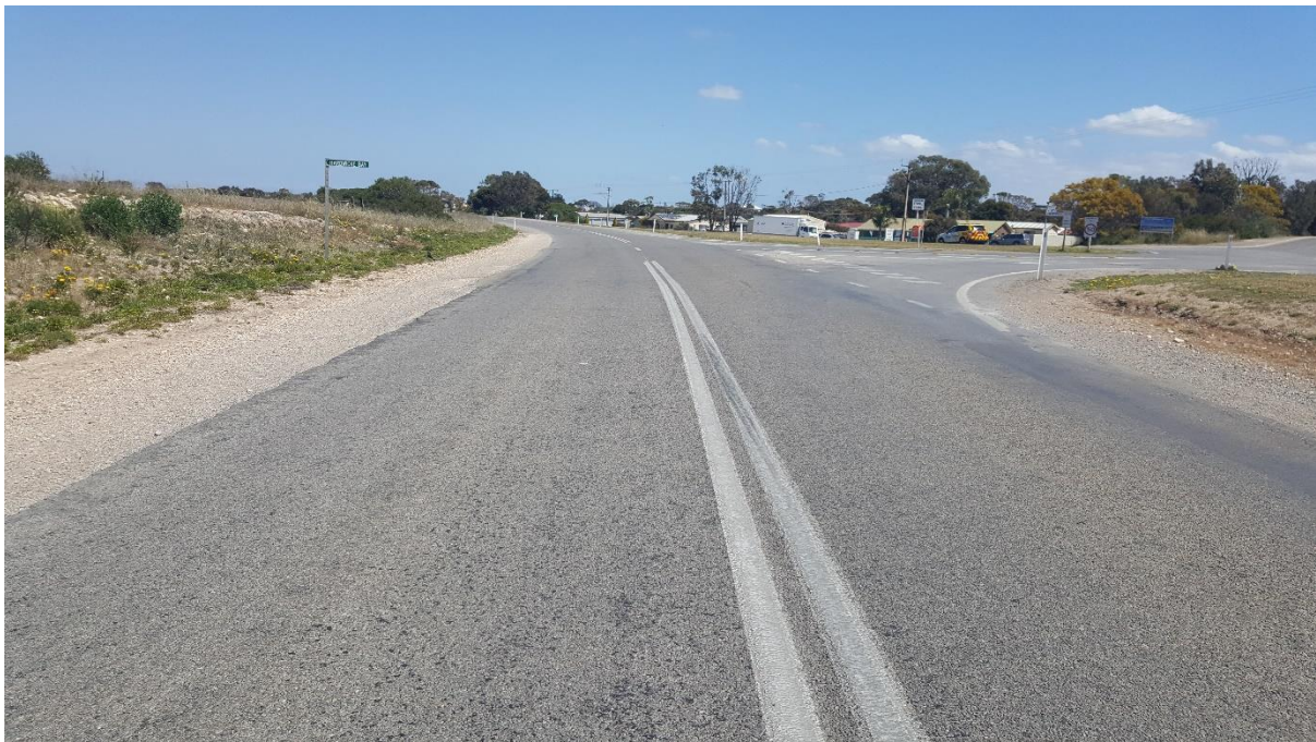
Poor sight distance turning right into Hardwicke Bay (North of the intersection, looking south)
