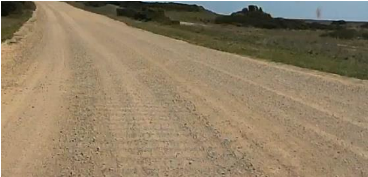
Corrugations on North Coast Road, and a build-up of loose surface material around a curve
