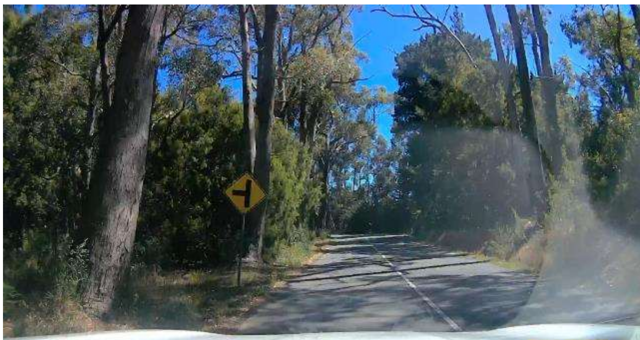
Figure 81: Roadside hazards and outdated intersection warning signage on Marble Hill Road.
