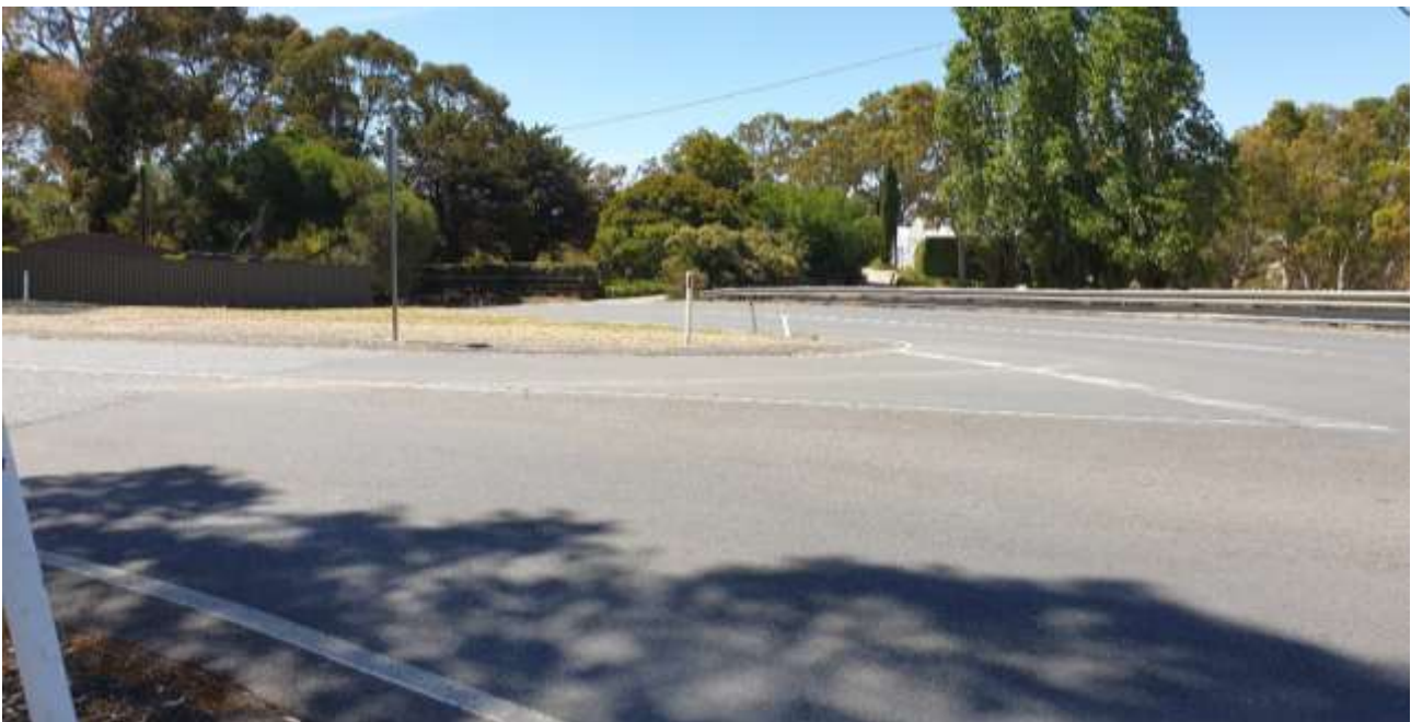
Figure 65: Poor sight distance at the intersection of North East Road and Lower North East road
