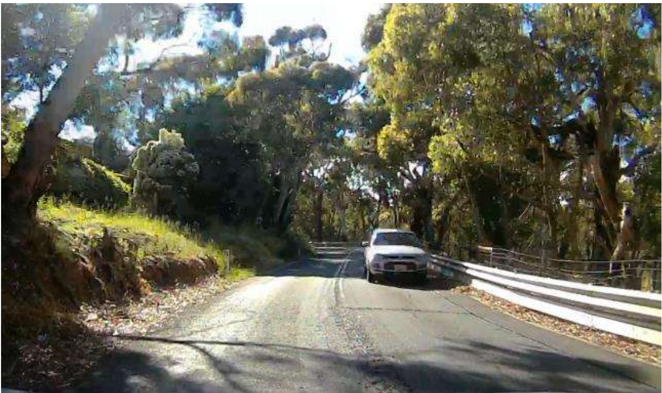
Figure 52: Deteriorated centre line marking and failing pavement on Greenhill Road
