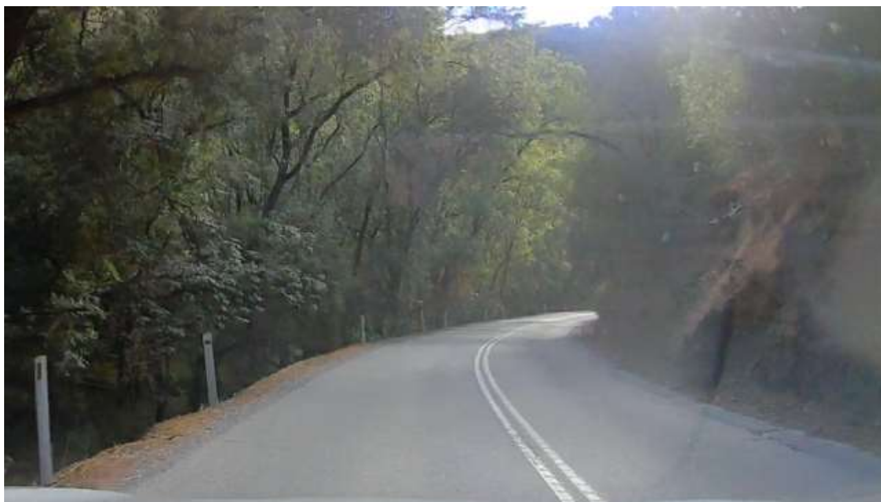
Figure 69 Example of a narrow section of Gorge Road with insufficient barrier protection
