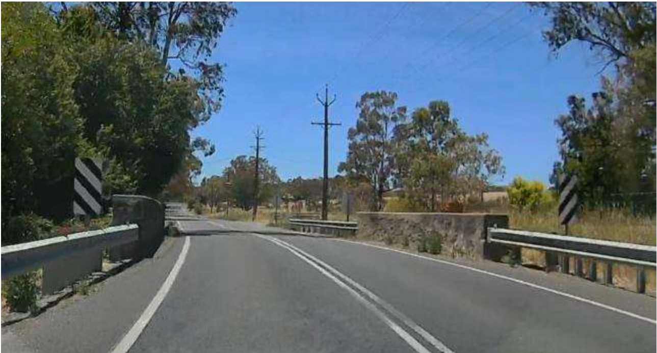
Figure 45: Narrow bridges are the most substantial geometric hazard on Onkaparinga Valley Road.
