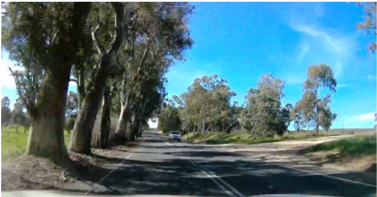
Figure 61: Exposed roadside hazards between Birdwood and Mt Pleasant
