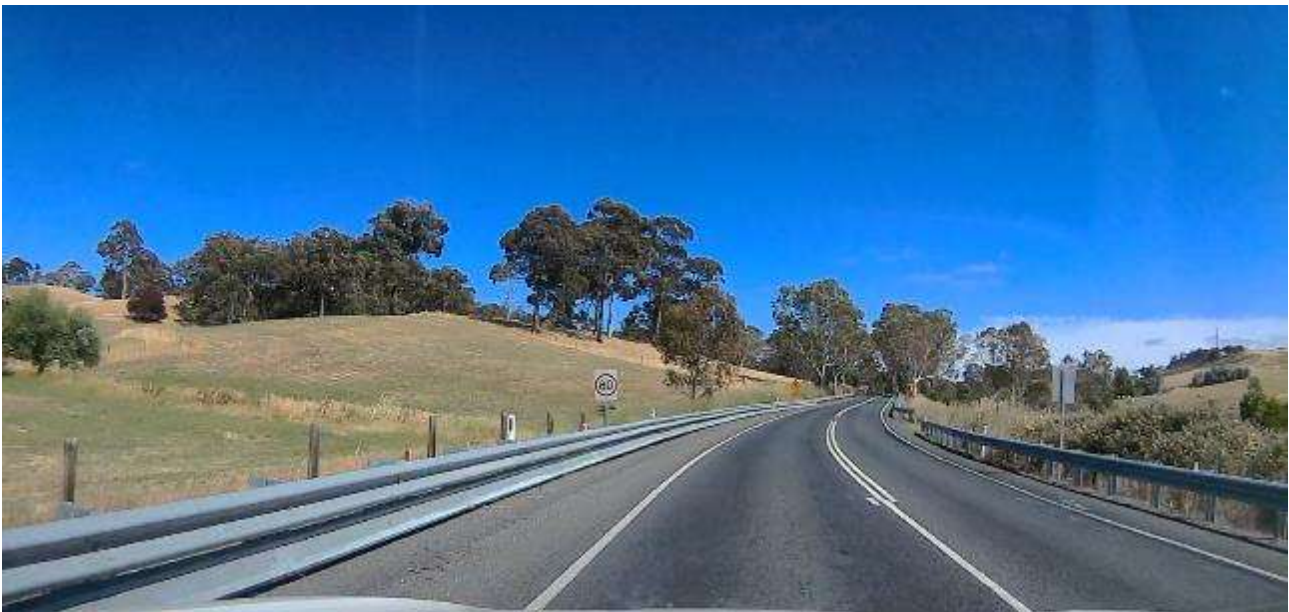
Figure 83: Wide sealed shoulders and motorcycle friendly barriers are typical safety treatments on Cudlee Creek Road
