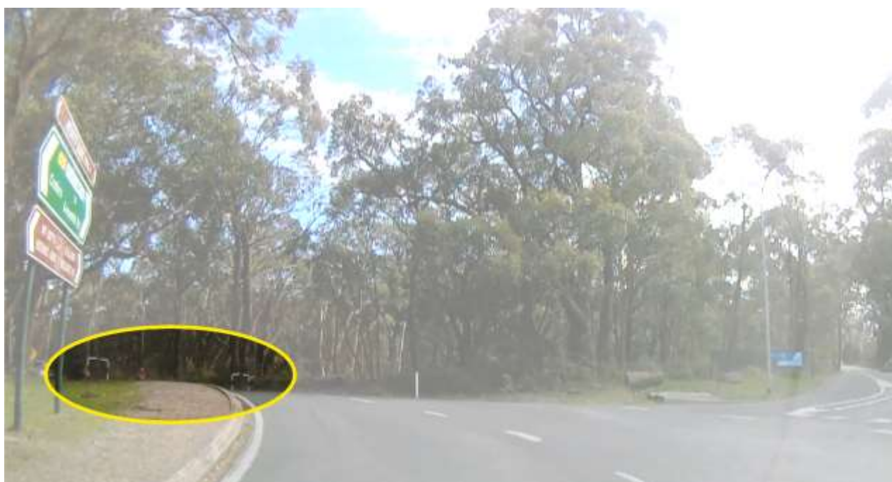
Figure 77: Pedestrian crossing point near Mt Lofty Summit obscured by horizontal and vertical road geometry
