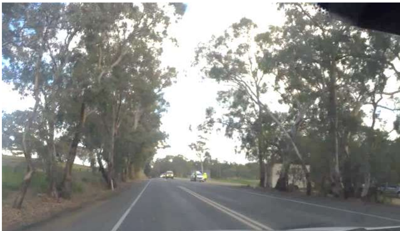
Figure 73: Cross section just south of Wistow with sealed shoulders, adequate carriageway width and exposed trees.
