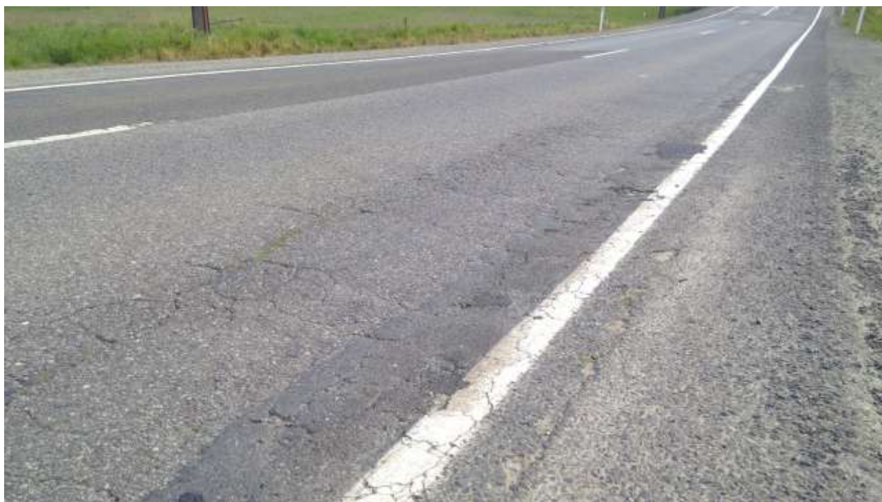
Figure 87: Typical pavement deterioration encountered along most of Piccadilly Road
