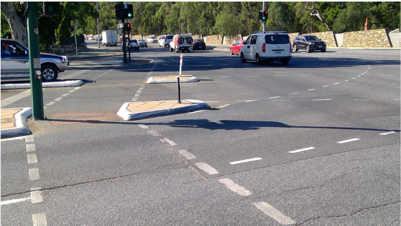
Pedestrians have minimal separation from turning traffic within the various refuges (Portrush Road refuge pictured)
