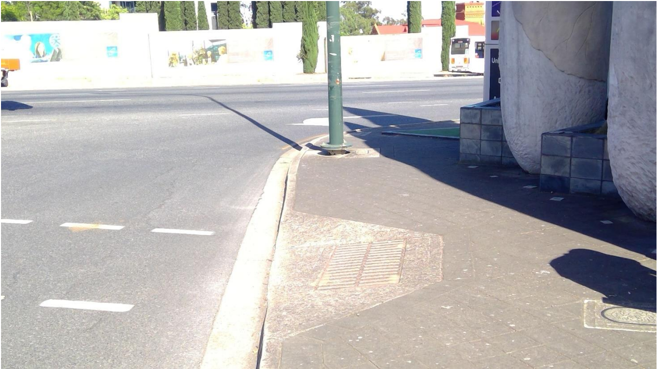
Approaching traffic is hidden from pedestrians at the crossing point on the Glen Osmond Road to Portrush Road slip lane
