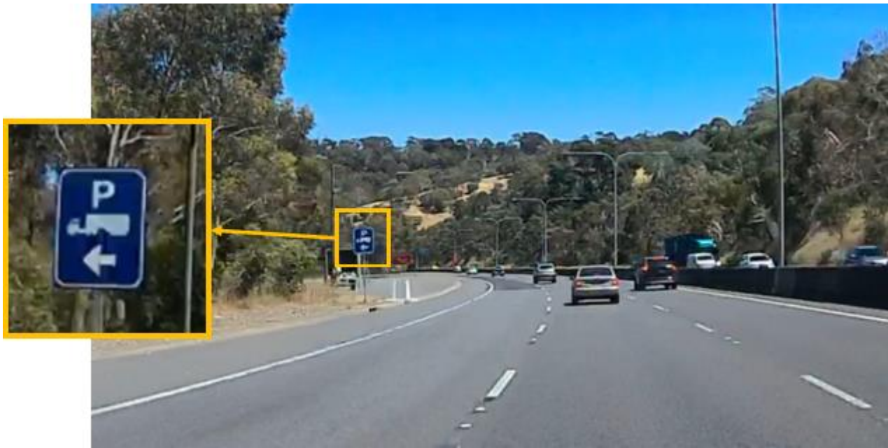
Only one sign identifies the truck parking/brake checking area west of the Heysen Tunnels
