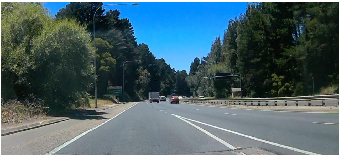
The length of the eastbound Crafers on-ramp creates difficulties for motorists entering the South Eastern Freeway
