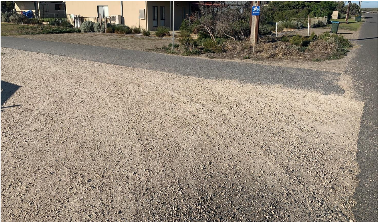
Figure 8: The gravel shoulder at the intersection with Andrew Avenue and Newell Avenue creates a rollover risk for cyclists
