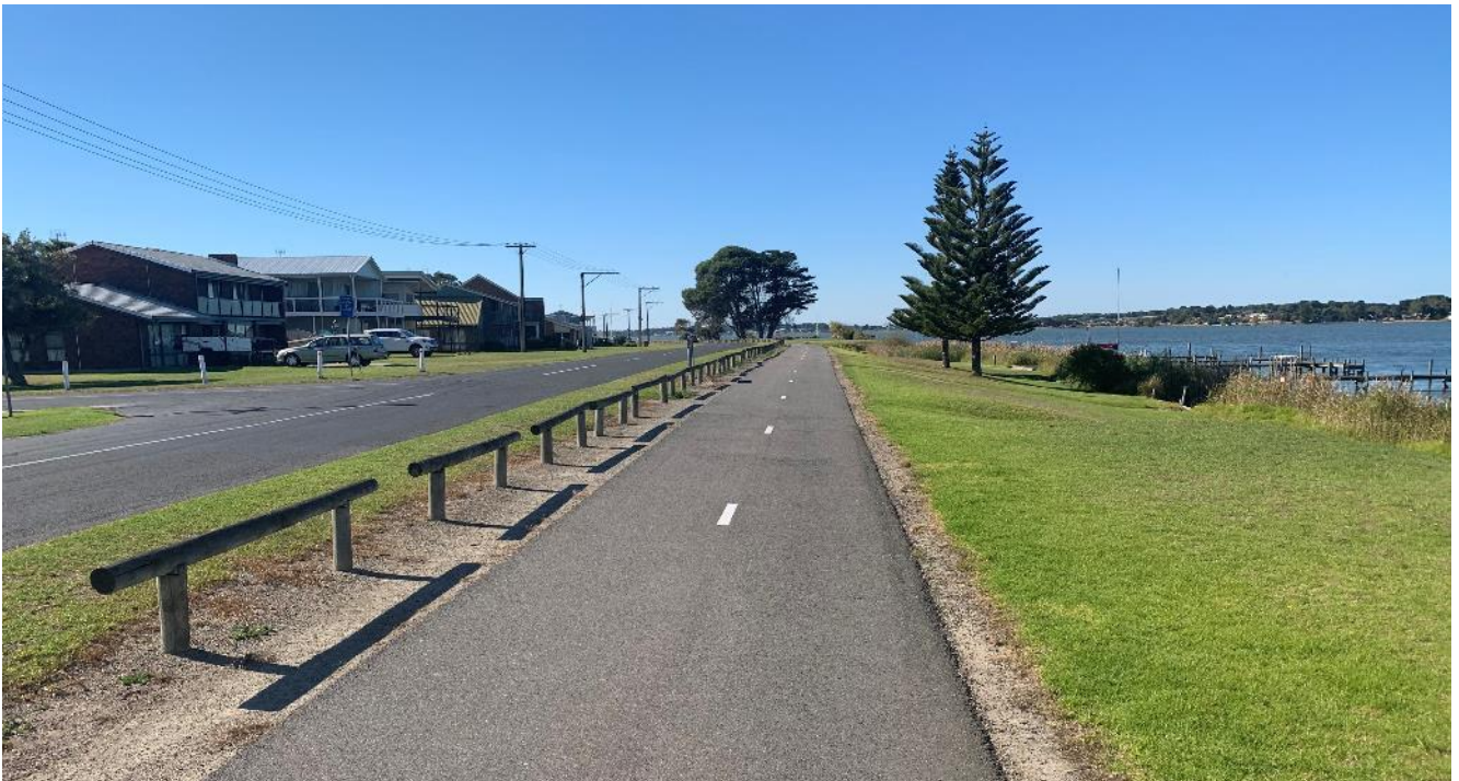
Figure 5: The Encounter Bikeway is constructed to a good standard in Goolwa North
