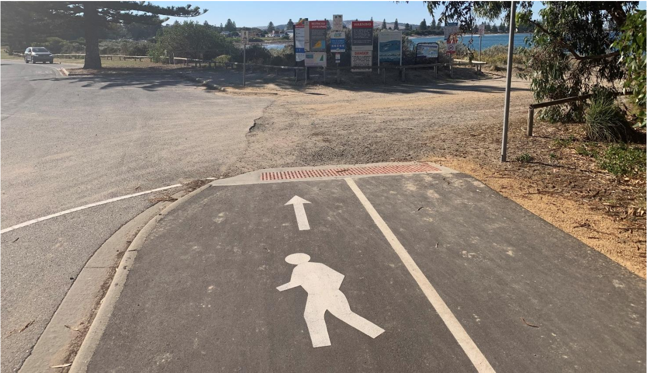
Figure 13: The wide path ends abruptly for eastbound path users at the beach access driveway in the Kent Reserve carpark
