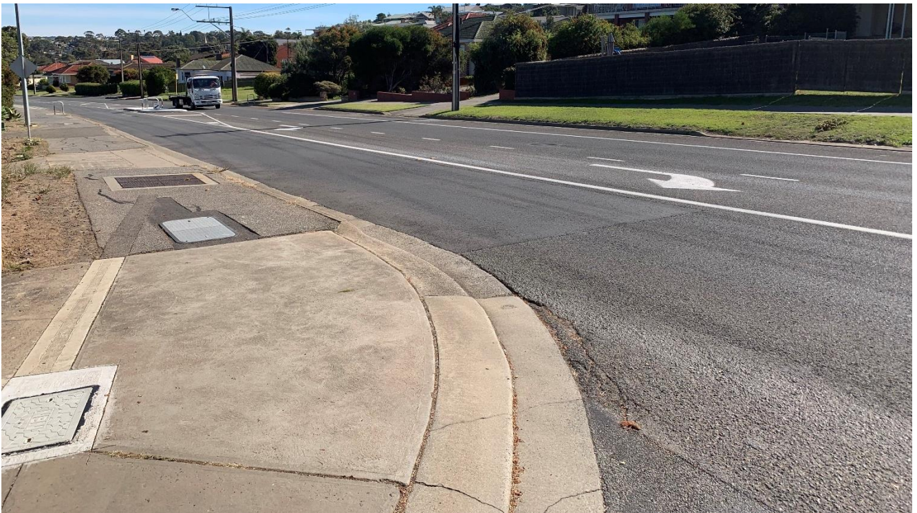
Figure 11: Hindmarsh Road in McCracken is an uncomfortable and hazardous cycling environment
