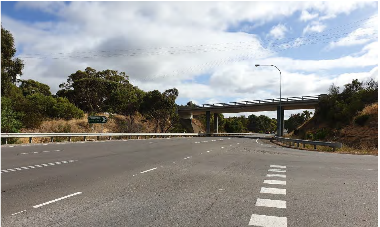
Figure 65: Sight distance to the north is obscured by the Greenhills Road bridge pylon
