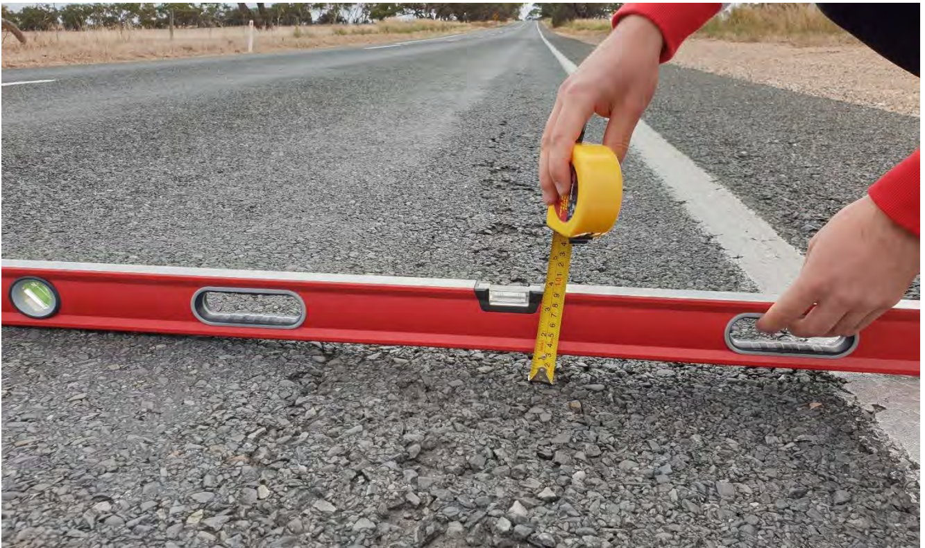
Figure 52: 30mm deep ruts and surface ravelling in Sandergrrove
