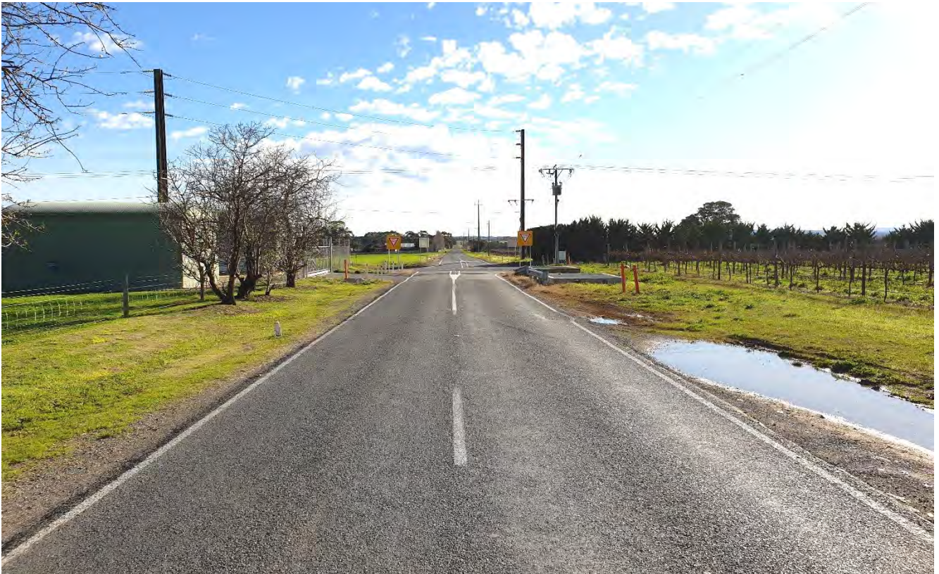
Figure 63: When approaching the intersection from the minor road approach, it can appear to drivers as though they are on a continuing road.
