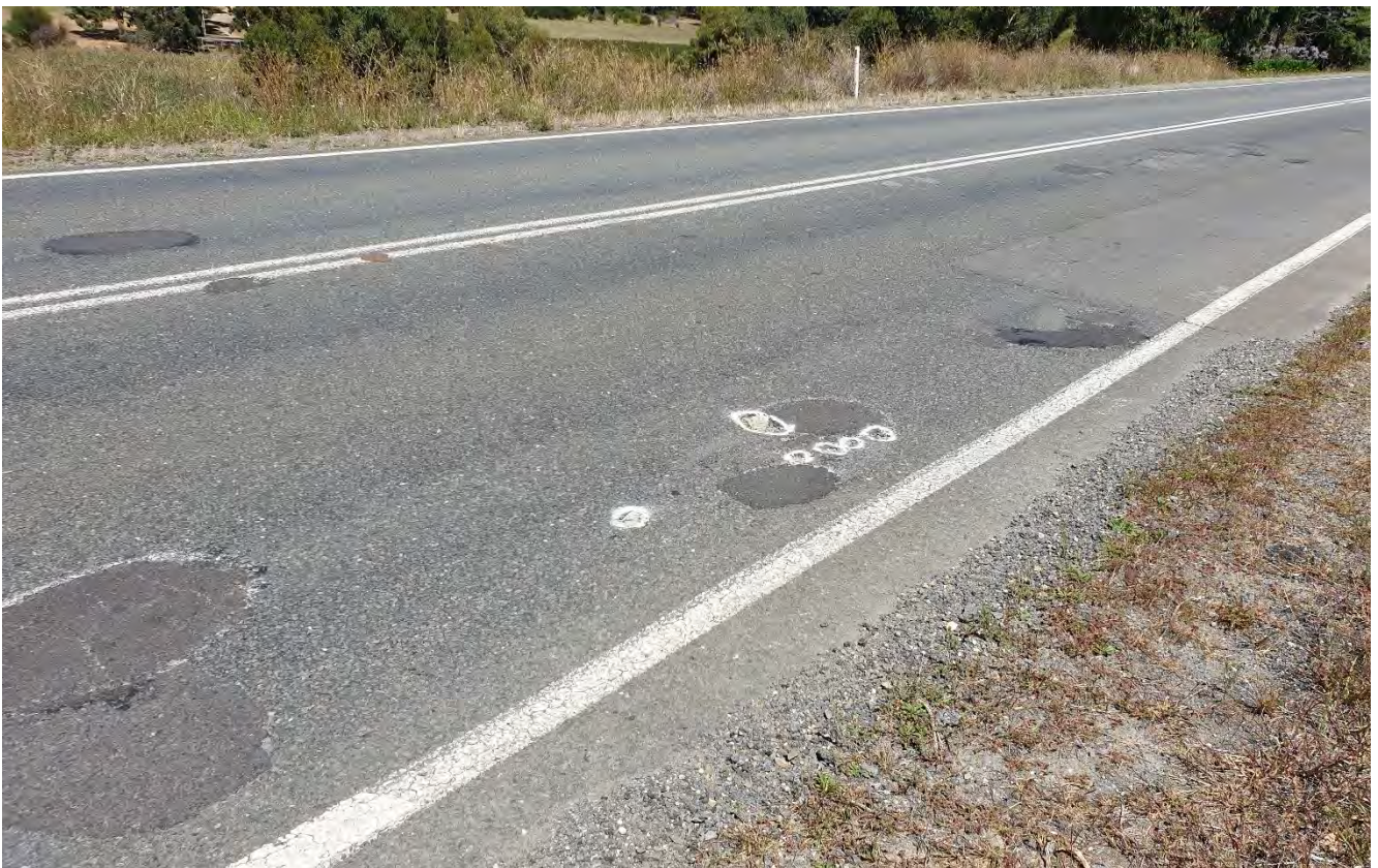
Figure 75: New potholes forming around recently repaired potholes.
