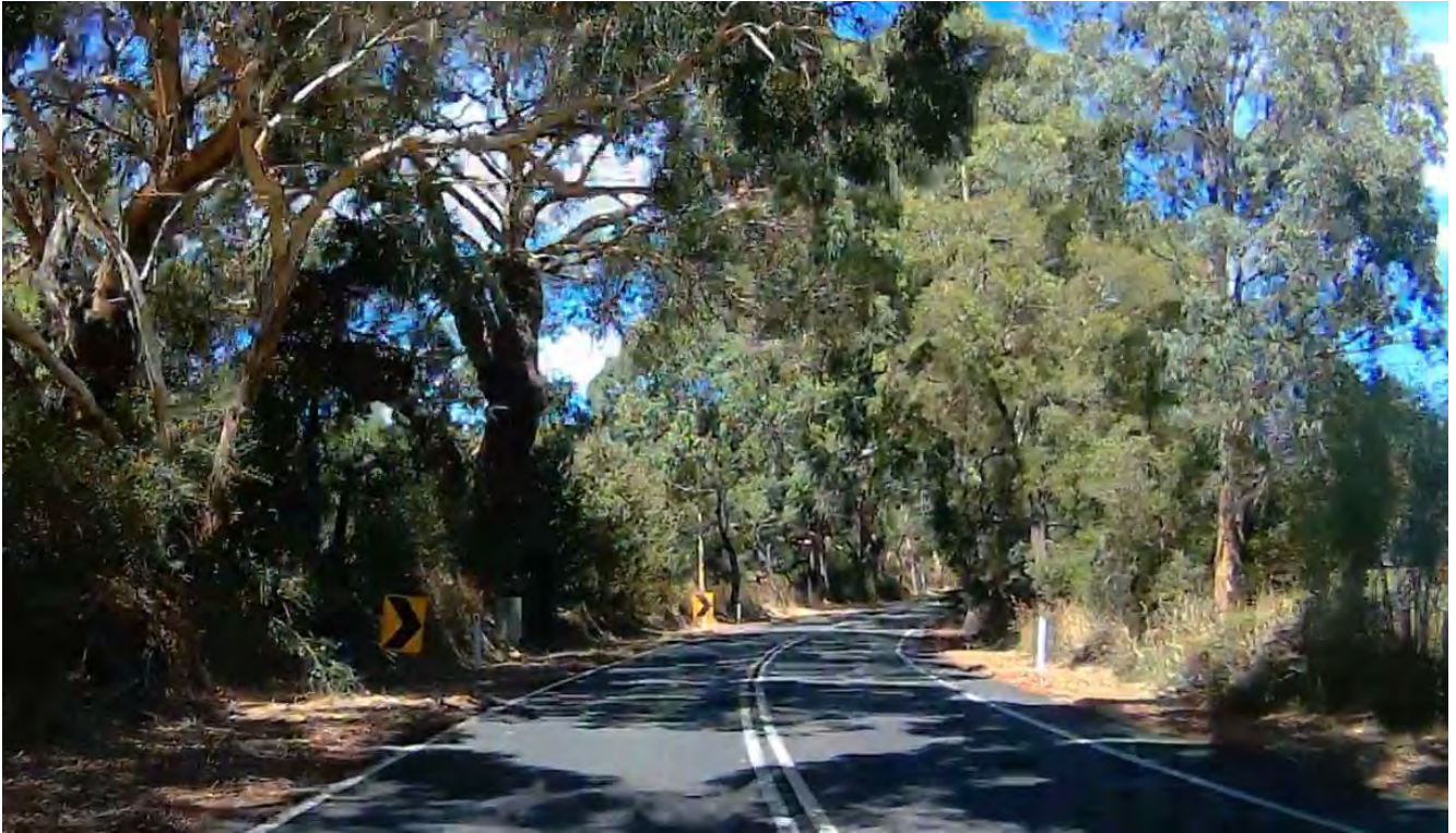
Figure 81: Large exposed trees on the outside of curves present a significant road safety risk on Bull Creek Road
