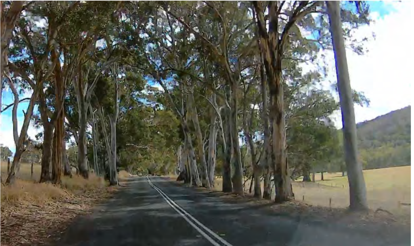
Figure 44: Trees on the roadside present the most significant hazard to users of Inman Valley Road
