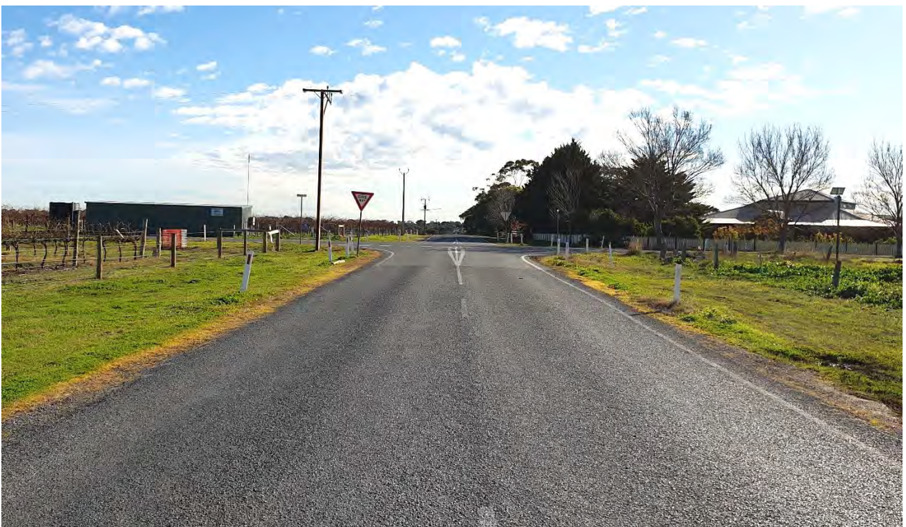
Figure 30: Although approaching a give way sign, there are few visual cues of the upcoming intersection other than signage (Intersection shown: California Road/Malpas Road, looking north on California Road)
