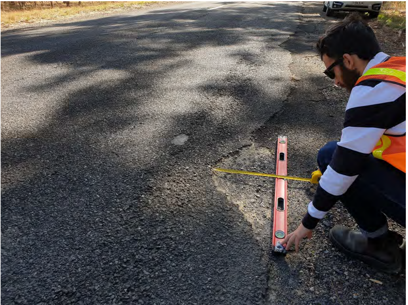
Figure 78: Edge break up on the eastern end of Range Road
