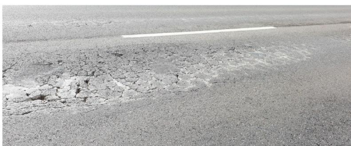
Fatigue cracking and rutting between McLaren Vale and Willunga.
