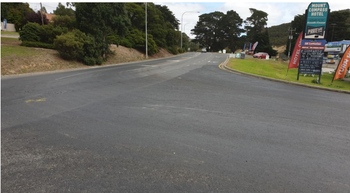
Figure 9: Faded line marking at the Intersection with Nangkita Road in Mount Compass
