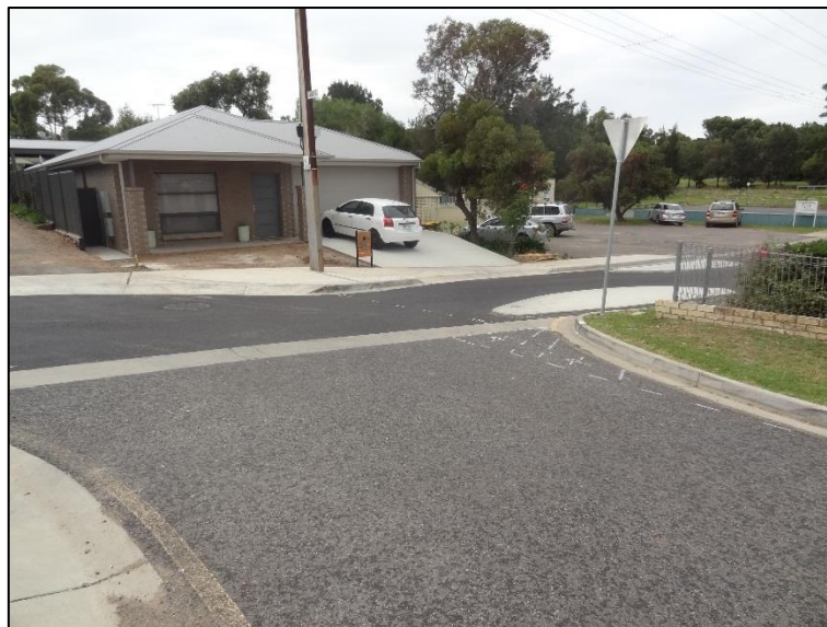
Figure 10 – Absence of centreline marking at Mill Street does not clearly indicate that the road continues to the left. Note – photo was taken during the first audit in March however centreline was absent during second audit in June.
