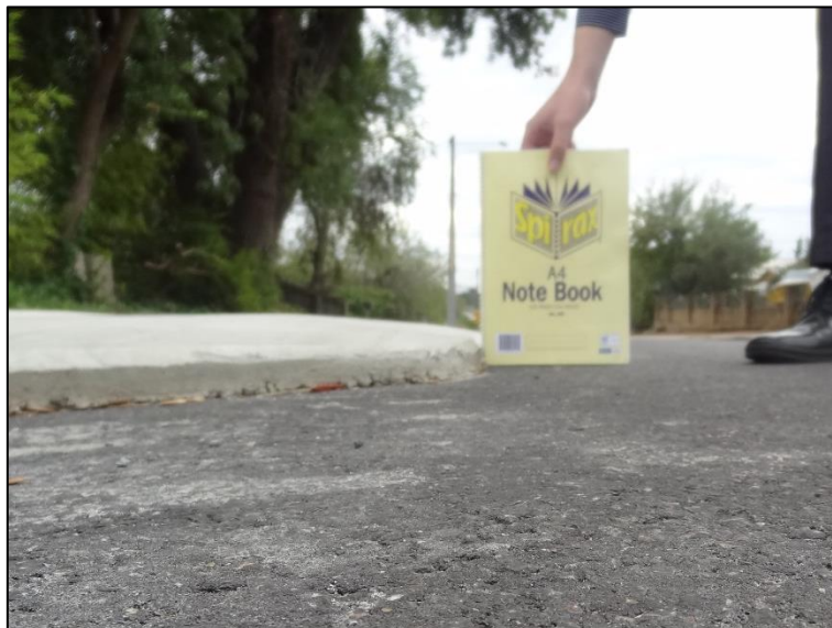
Figure 6 – Example of a shallower island, almost half the height of that shown in Figure 7.
