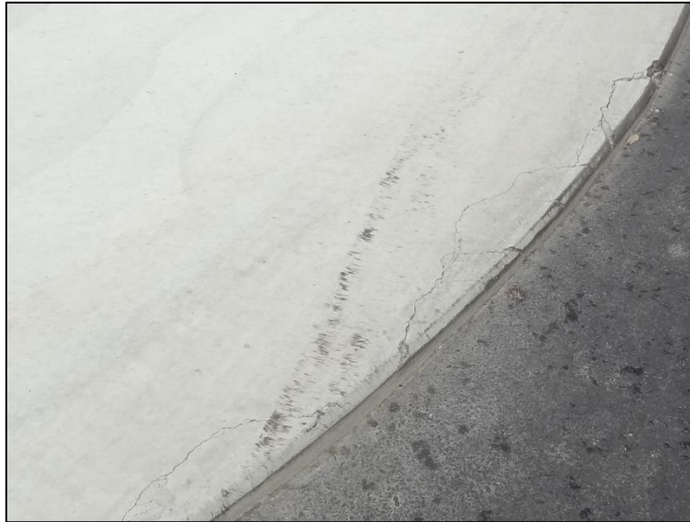
Figure 5 – Concrete islands are already starting to crack and break away at the edges.
