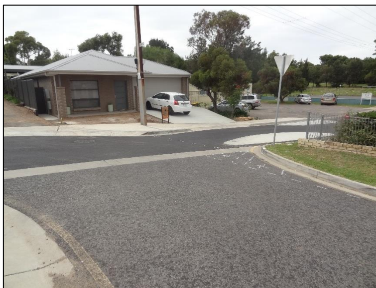
Figure 2 – Chicane at the intersections of Mill Street (pictured) and Olive Street could cause safety and traffic issues for vehicles turning into the chicane while vehicles approach from the opposite direction.
