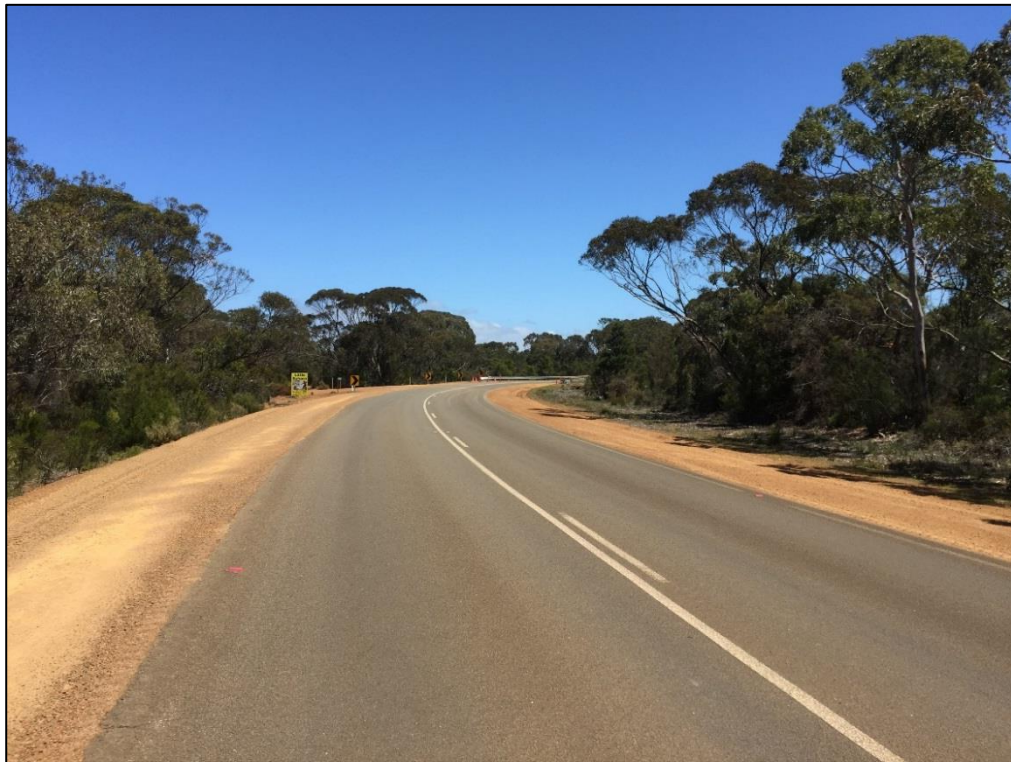
Figure 4 – CAMs do not adequately inform the approaching driver of the radius of the curve. Distinctive arrow on ‘Little Sahara Dunes Complex’ entrance sign should be incorporated to provide further clarification to approaching drivers.
