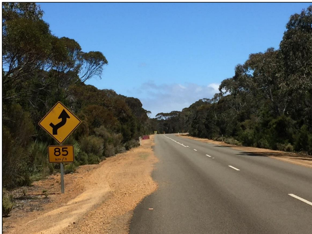
Figure 2 – Speed advisory sign back too far from the corner and should be relocated. No advance warning of major tourist attraction so vehicles have adequate time to slow down and passing traffic aware of the driveway and possible traffic movements.
