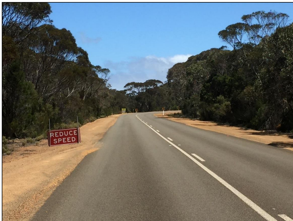
Figure 3 – Sequencing of signage could result in the driver not realising the radius of the approaching curve and that 'Reduce Speed' pertains to the Little Sahara Dunes Complex access driveway rather than the curve.
