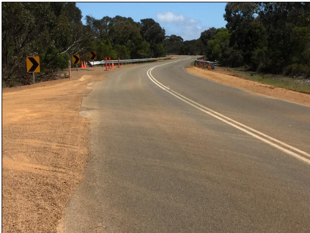
Figure 6 – The shoulders are unsealed and present a risk of vehicles skidding should the vehicle drift out of the traffic lane.
