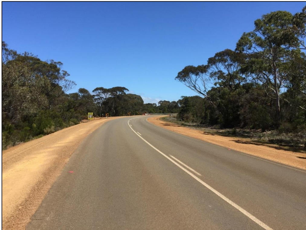
Figure 5 - Faded edge line marking to be reinstated.
