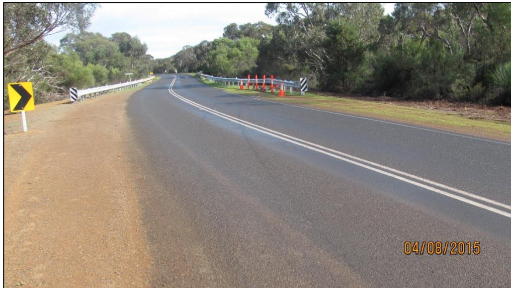
Figure 7 – The crash barrier commences late into the curve and provides limited protection to vehicles that drift off the road at the curve transition.
