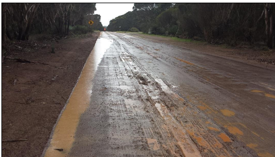
Figure 2 – A poor surface when wet results in reduced skid resistance.
