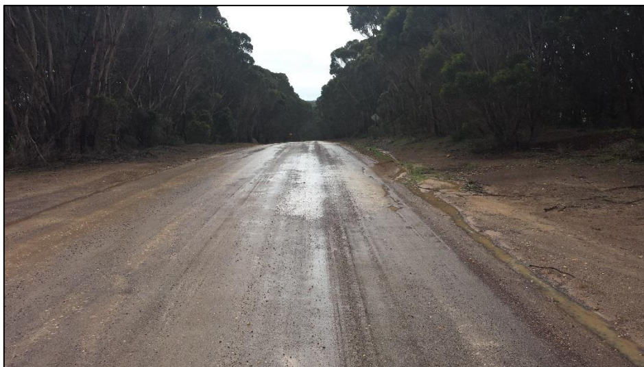
Figure 5 – Sight distance (northbound) from Moffatt Road is restricted by a crest on Willson River Road.
