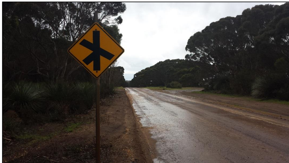
Figure 4 – Intersection warning sign is non-standard and in close proximity to the intersection.
