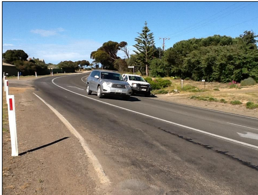
Figure 2 –Steep geometry over extended lane width created sight difficulty for entering traffic. (Note excavation depth into the opposite embankment)
