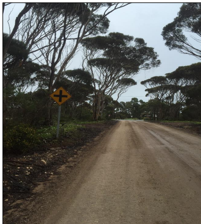
Figure 8 - Tinsmith Road approach- Cross road sign obscured by vegetation from further back.
