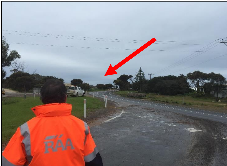
Figure 3 – Sight Distance- the vegetation indicated obstructs long range sight distance. On observation, drivers tend to hold further back from the Give Way line in order to optimise their view of oncoming traffic from Kingscote.
