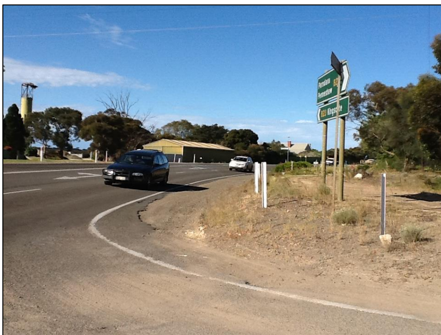
Figure 5 -The resultant embankment and relocation of signage associated with the works to increase the lane width on Playford Highway restricts sight distance to the east from Tinsmith Road.
