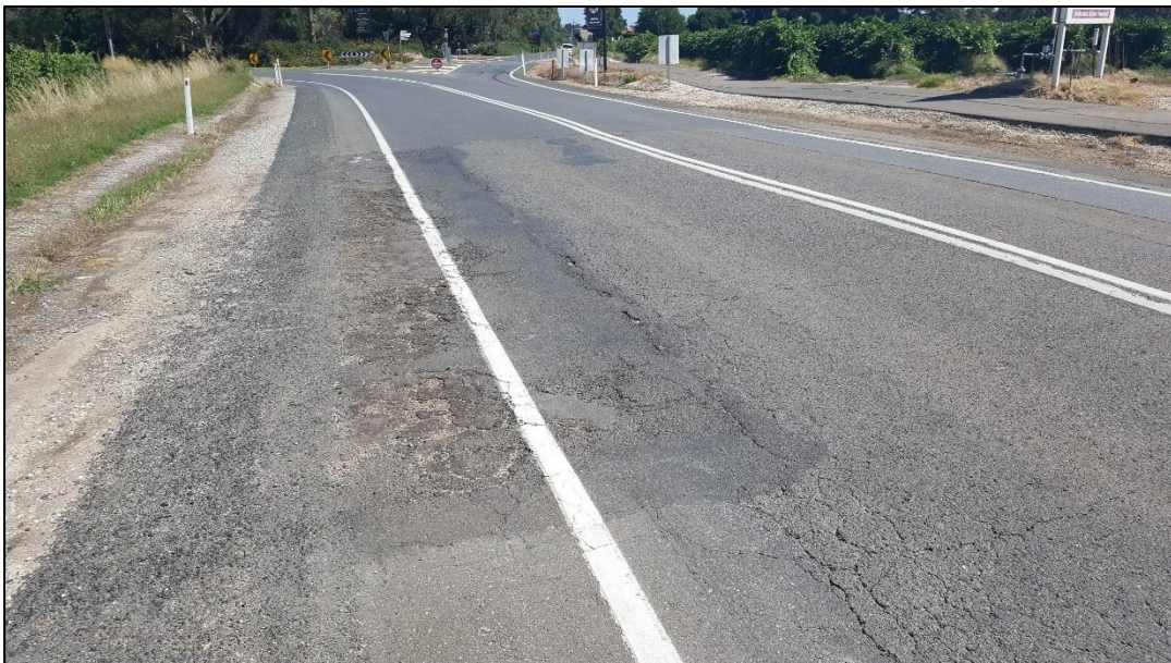
Figure 7 – Pavement deterioration.
