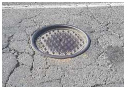
Pit cover opposite Stephenson Ave
