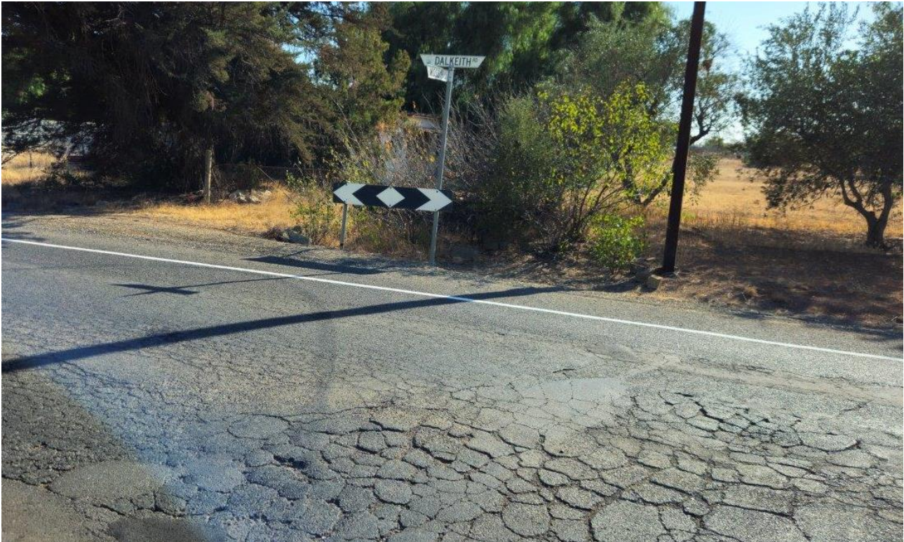
Figure 26: Cracked road surface at the intersection with Moss Road, Kudla (March 2025)
