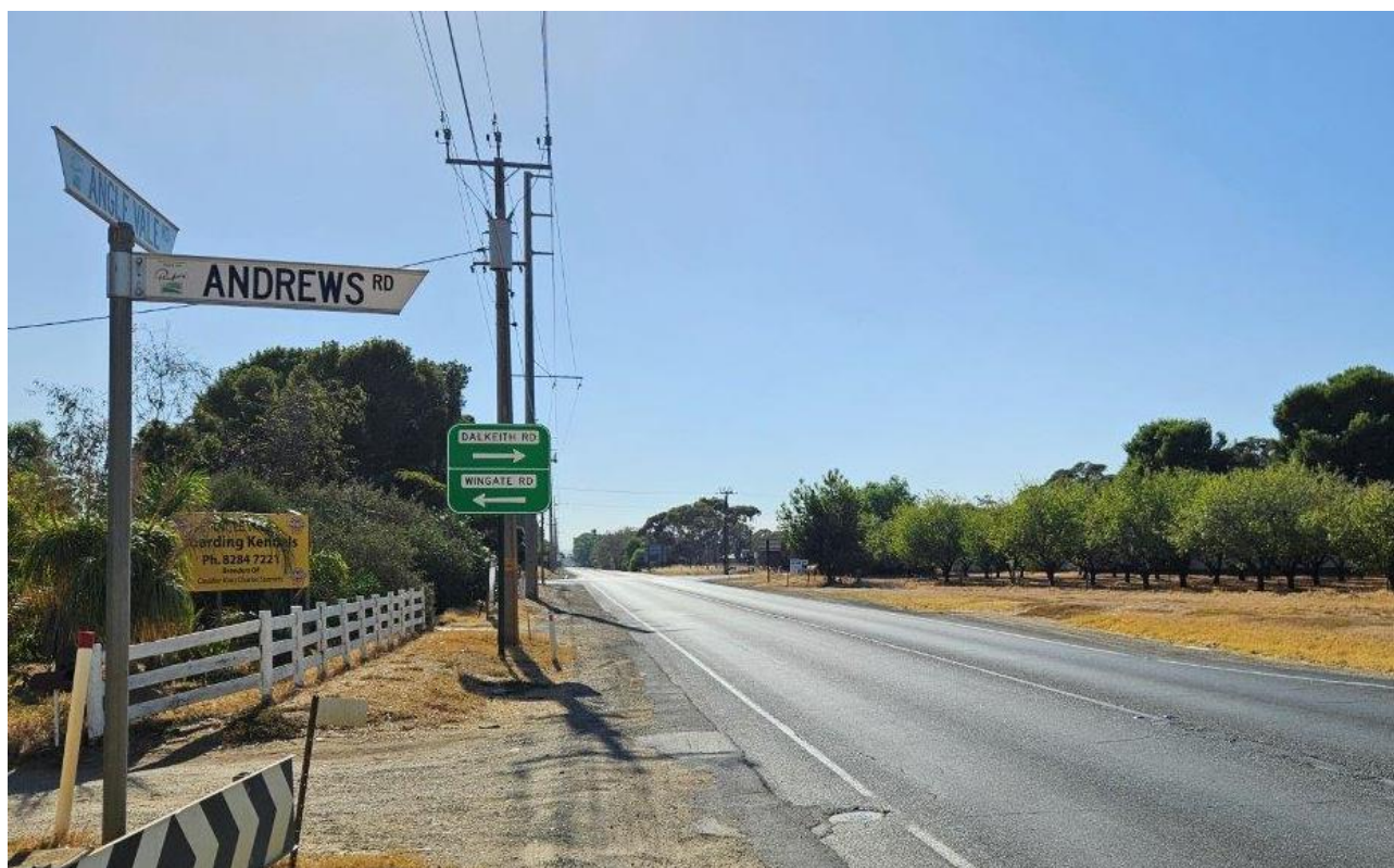
Figure 87: The two closely spaced intersections were highly raised for high traffic and lack of turning lanes
