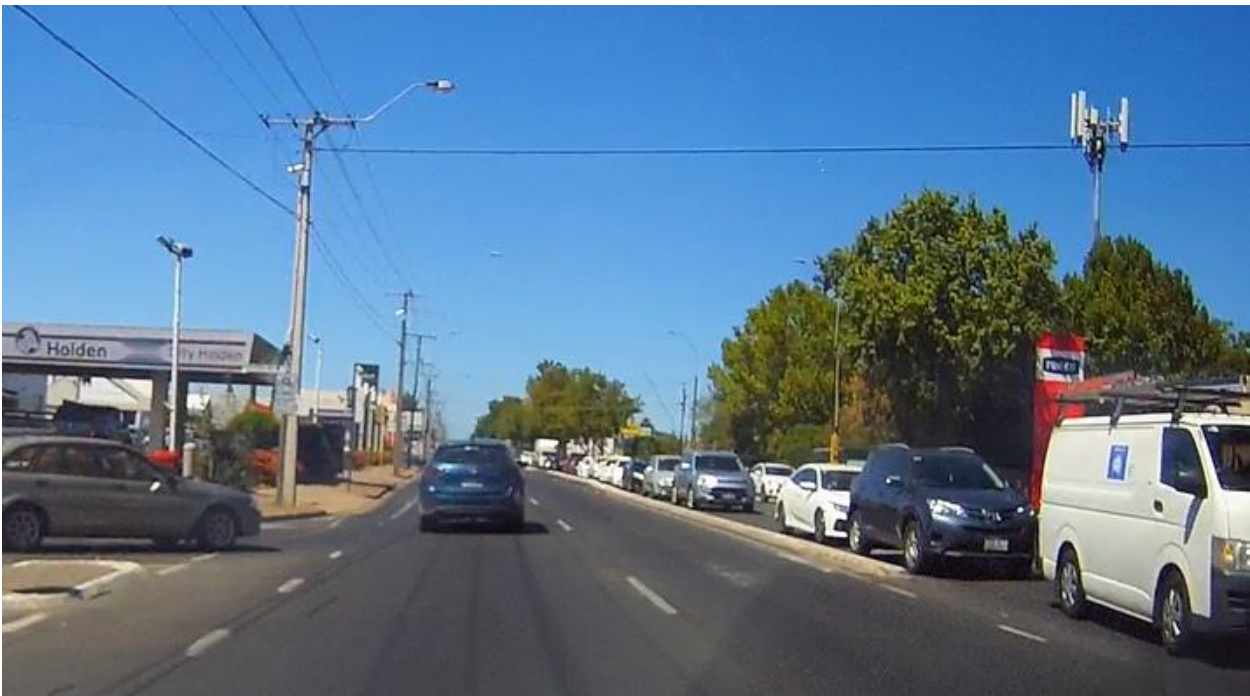
Figure 38: Long queues to turn right onto Fosters Road from North East Road extend beyond the channelised turn lane
