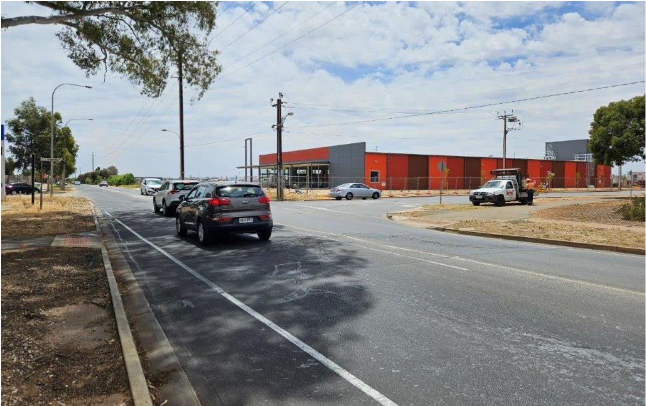
Figure 85: Cars turning right on to Andrews Road blocked through traffic on Curtis Road towards the Northern Expressway before a short channelised right turn lane was added in December 2024.
