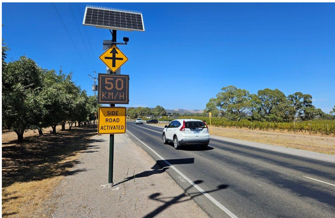
Figure 58: The RJAWS-Lite system installed on Main Road sets a 50km/h advisory speed when a vehicle is detected approaching from the side road (Malpas Road)
