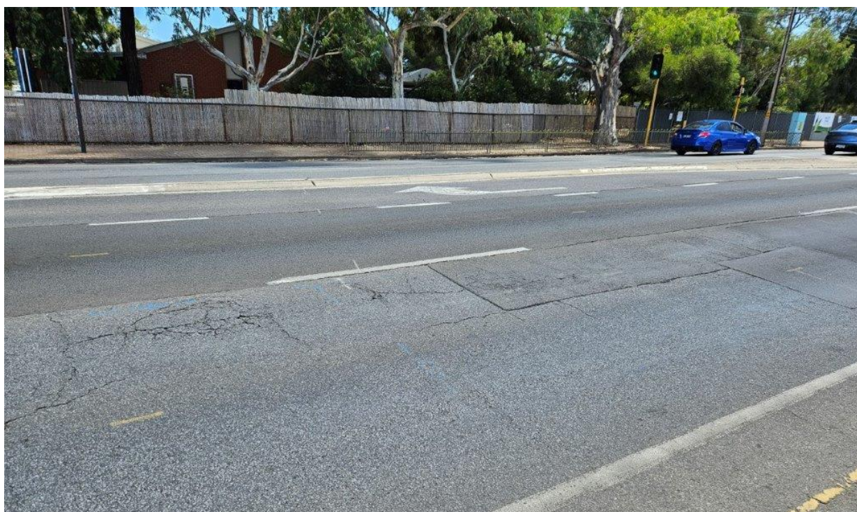
Figure 45: Cracking and multiple patches between Second Ave and Third Ave, Park Holme (Photo: December 2024)
