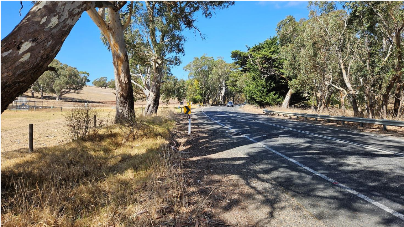
Figure 53: Narrow lanes, tight geometry and hazardous roadsides are all present on Main South Road
