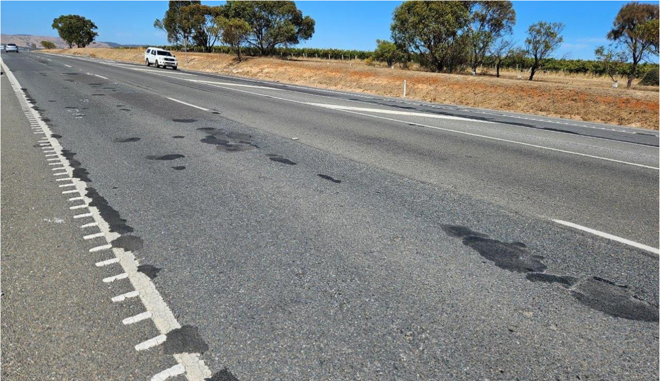
Figure 52: Potholes, rutting and undulations in the southbound overtaking lane between McLaren Vale and Willunga (photo March 2025)
