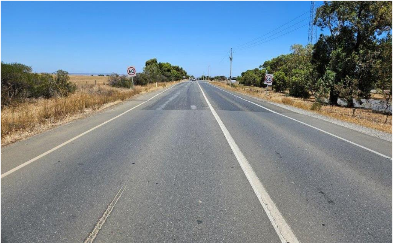
Figure 76: Undulations and deteriorating surface immediately north of Roseworthy (Photo: RAA, January 2025)
