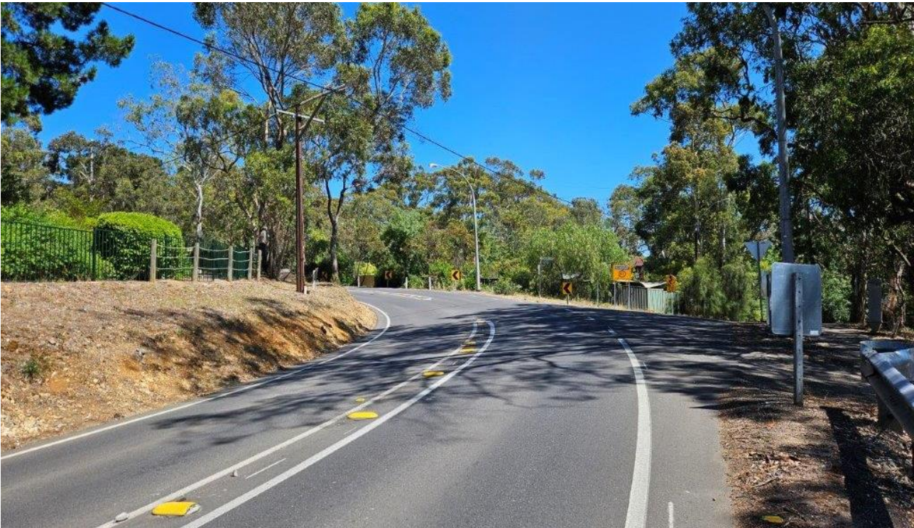
Figure 104: The embankment on the inside of the curve restricts visibility of opposing traffic when turning right onto Sturt Avenue
